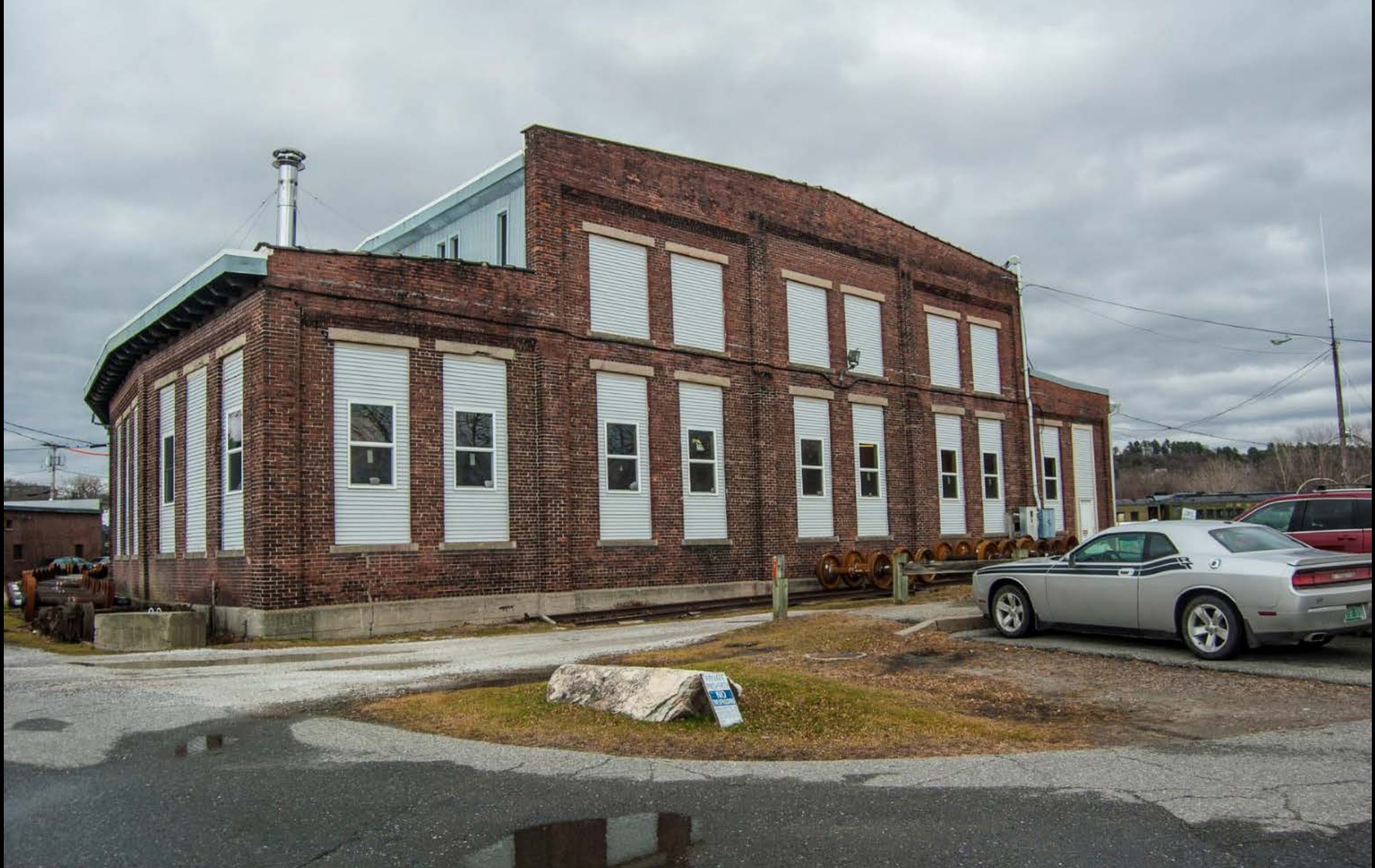
Photo 1. View looking north/northeast at HD #1b Railroad Engine Roundhouse.
