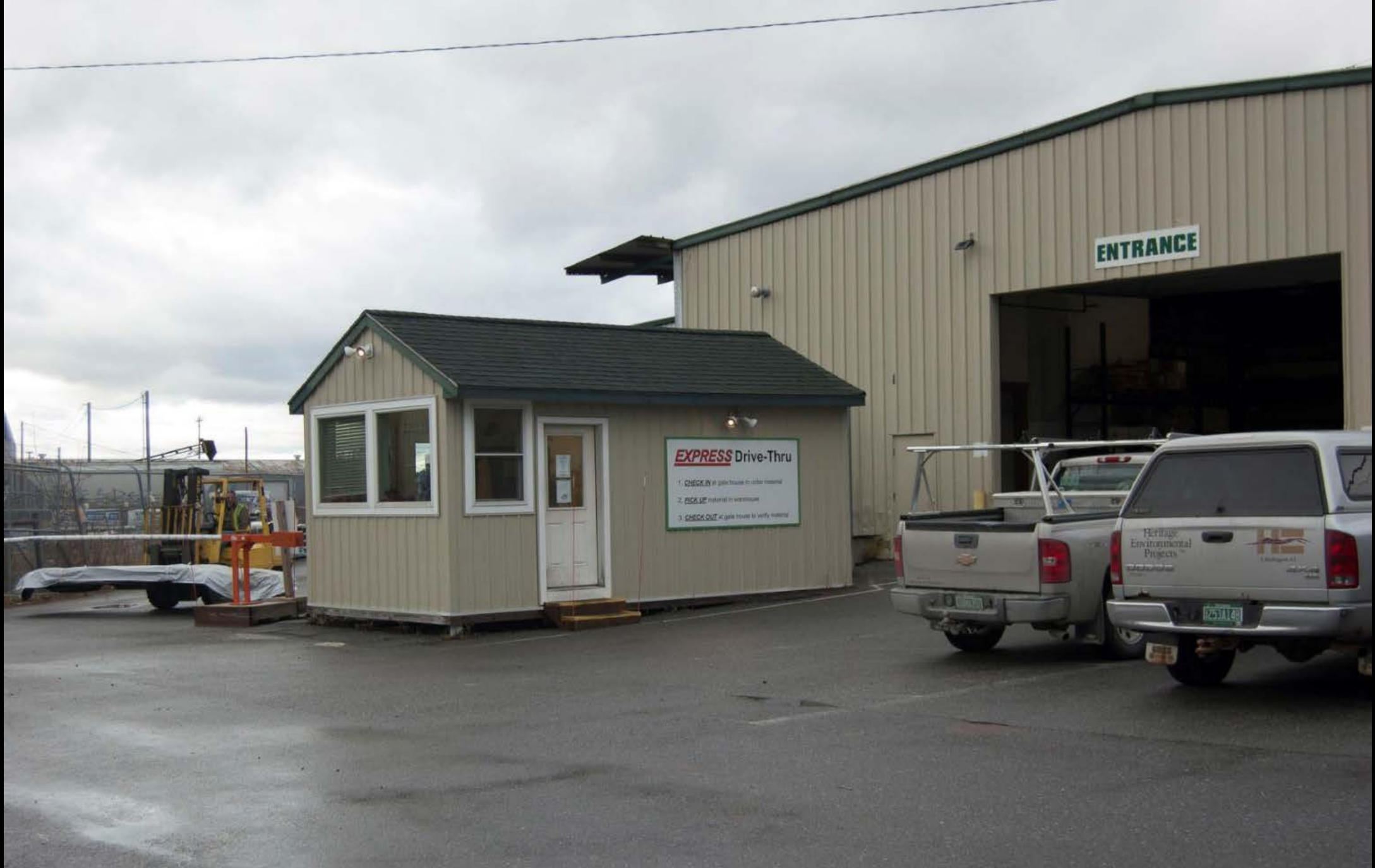
Photo 18. View looking west at HD #9a Shed.
