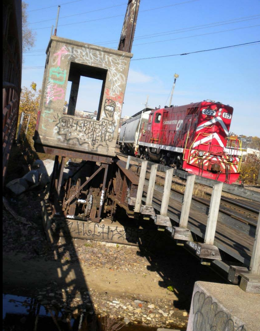
Photo 52. View looking north at HD #22 Drawbridge.
