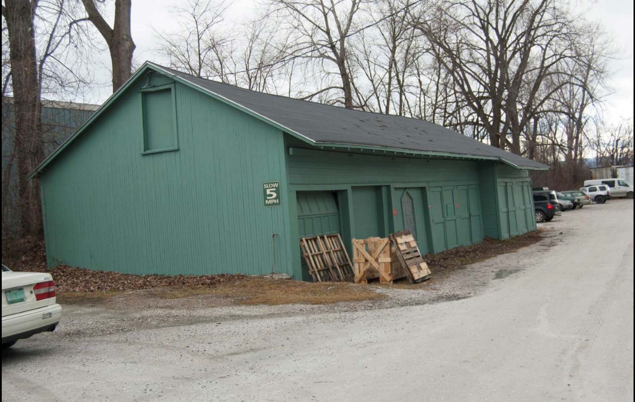
Photo 37. View looking west at HD #17a Wagon Shed.
