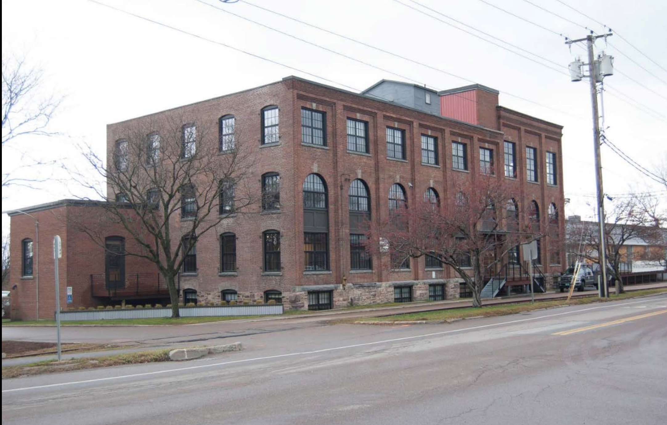
Photo 43. View looking northwest at HD #19 Malted Cereal Company.
