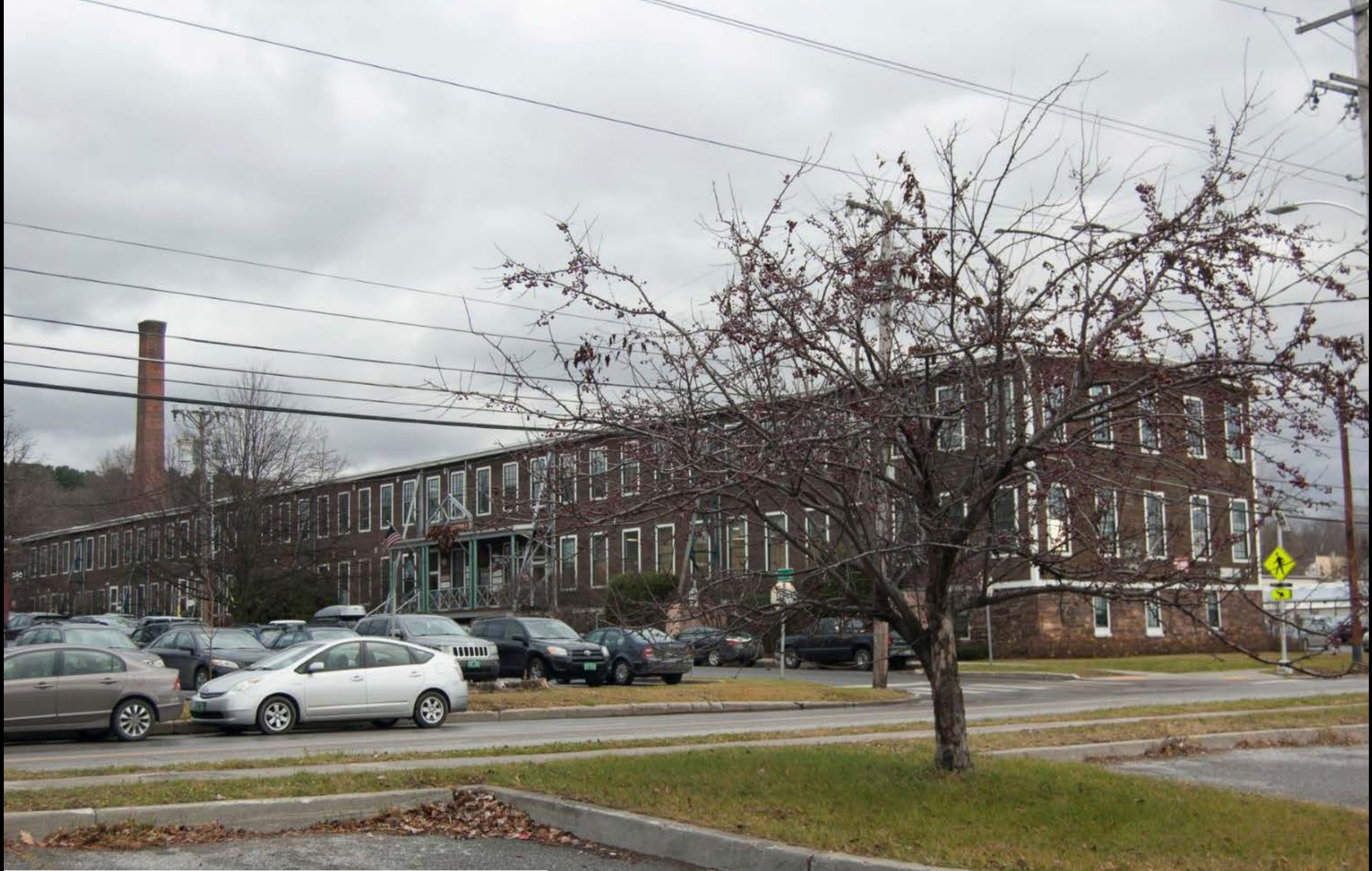
Photo 23. View looking southeast at HD #11 Kilburn and Gates.
