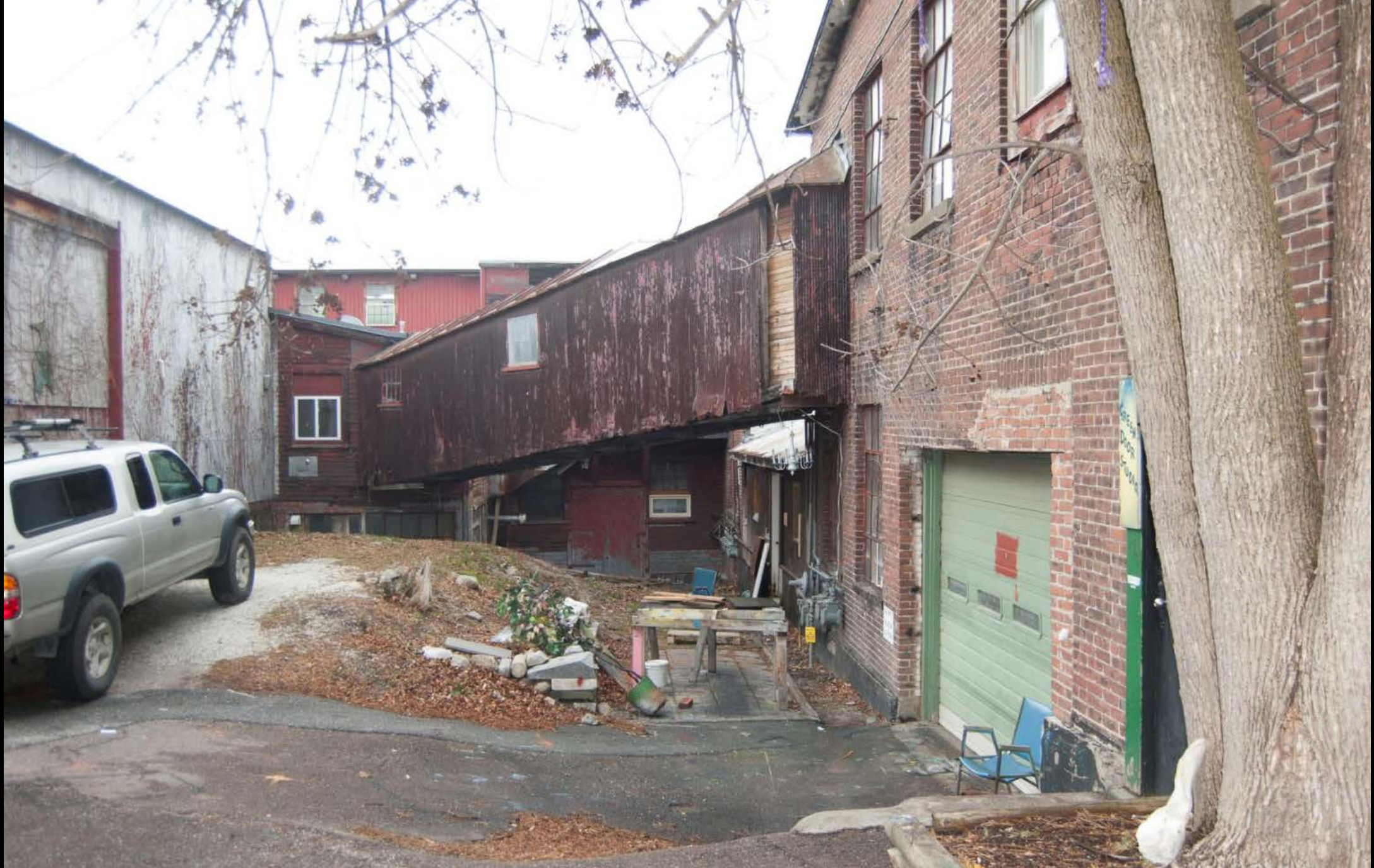
Photo 49. View looking west at rear of HD #20 E.B. and A.C. Whiting Company.
