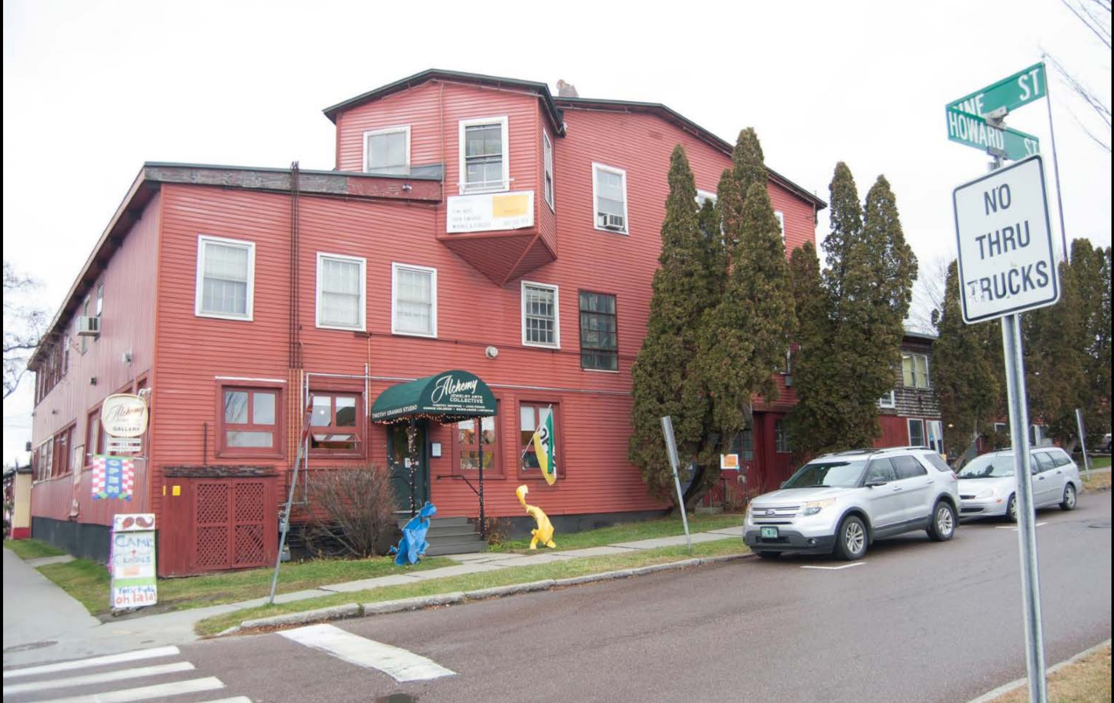
Photo 50. View looking north at HD #20 E.B. and A.C. Whiting Company.
