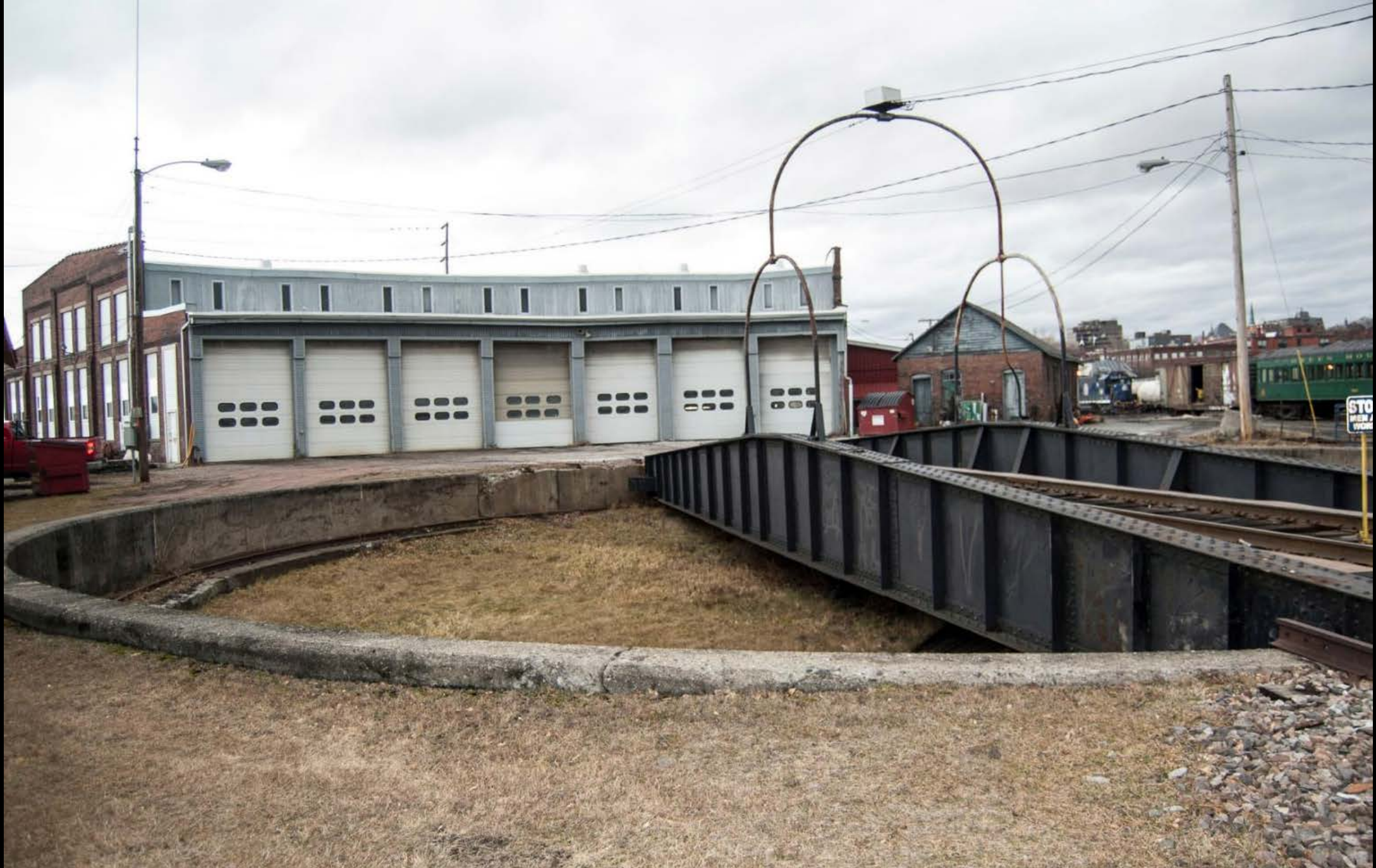
Photo 8. View looking north/northwest at HD #1c Turntable, HD #1b Railroad Engine Roundhouse, and HD # 1d Pumphouse/Boiler Room.
