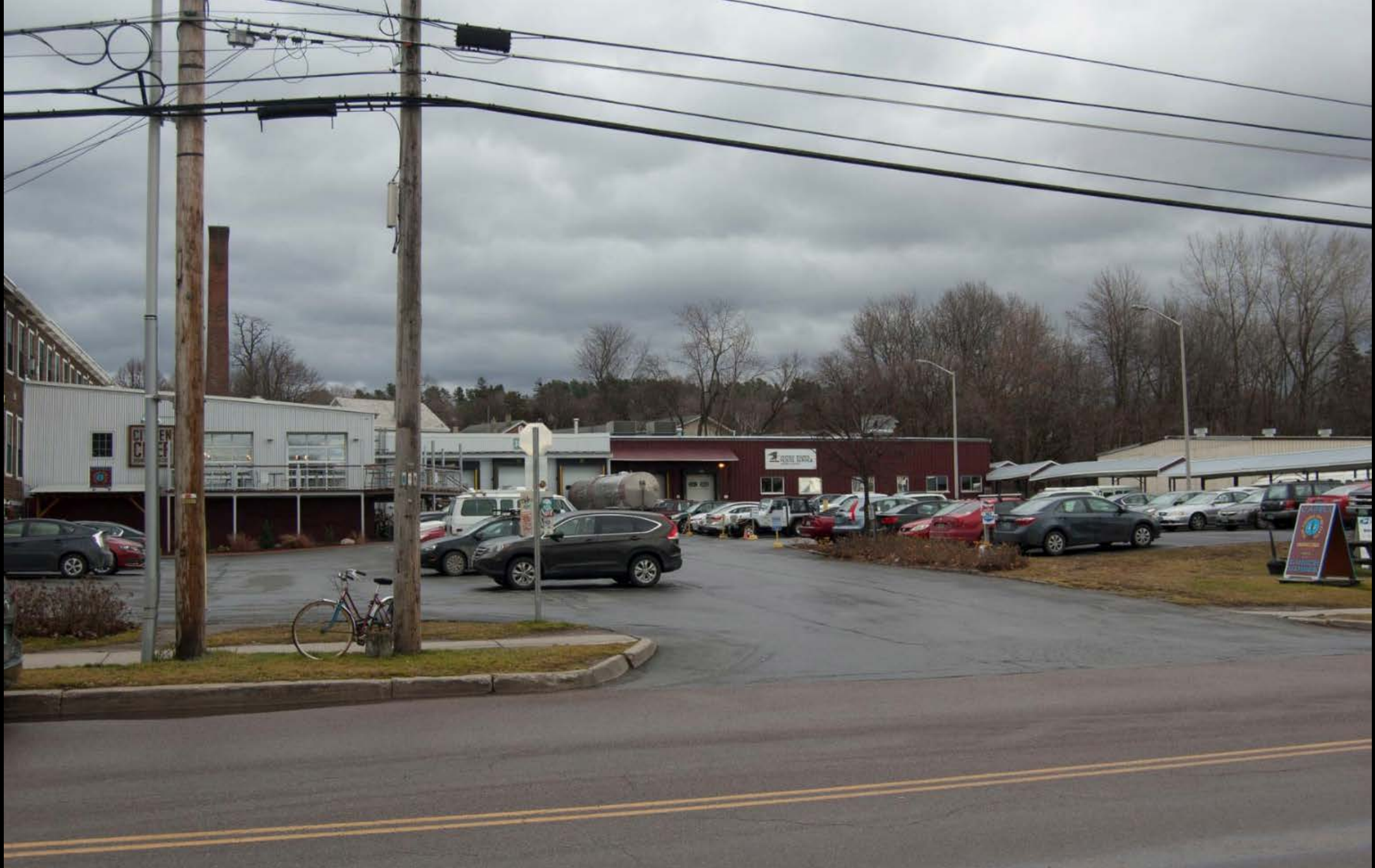
Photo 27. View looking east at additions on south wall of HD #11 Kilburn and Gates.
