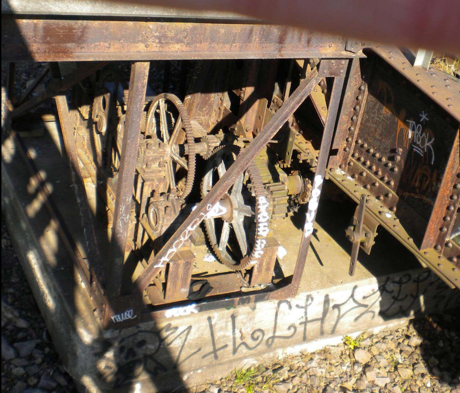
Photo 53. View looking north at HD #22 Drawbridge, detail of raising/lower mechanisms.
