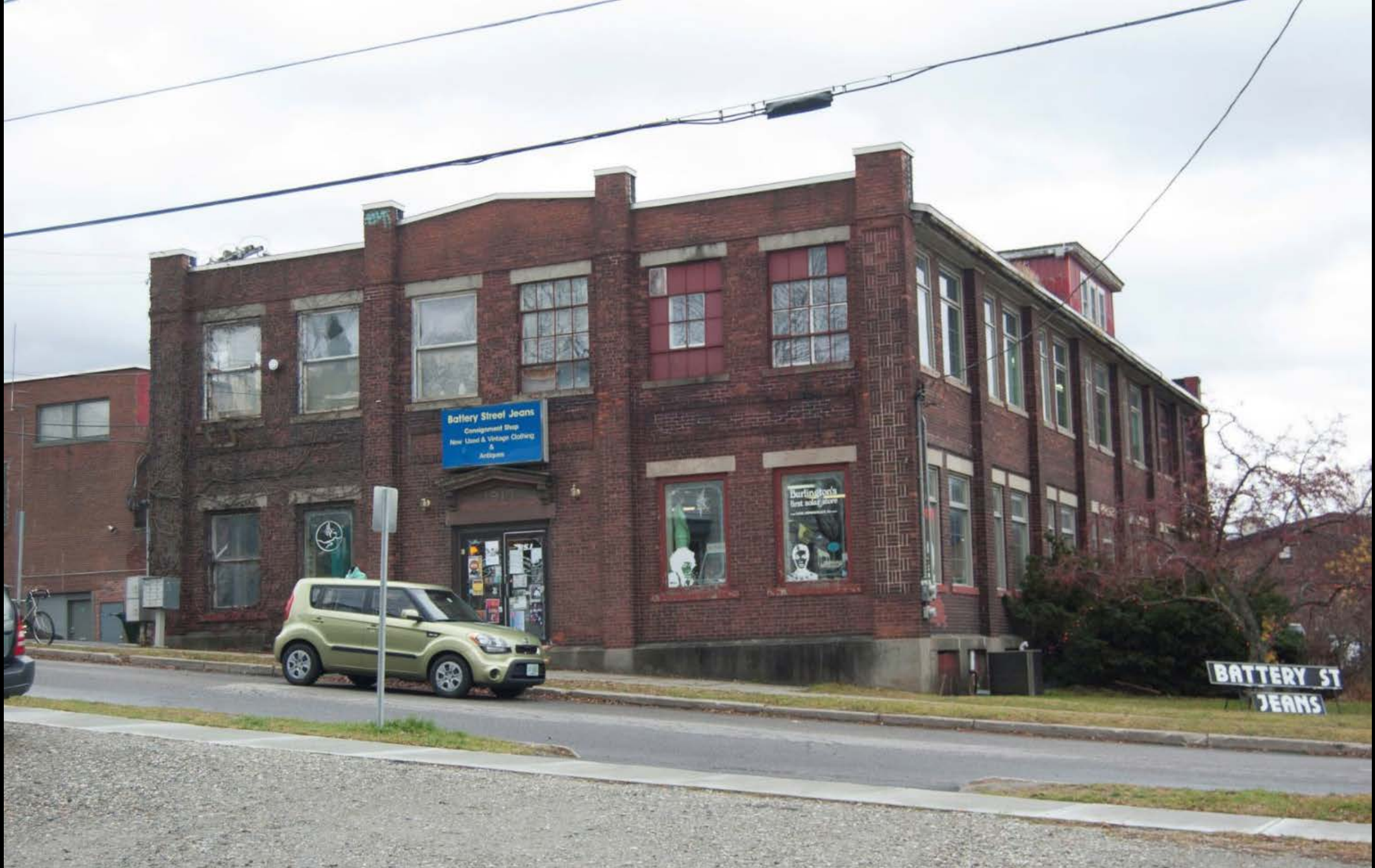
Photo 33. View looking south across Marble Avenue at the north façade of HD #15 Welsh Brothers Maple Company.
