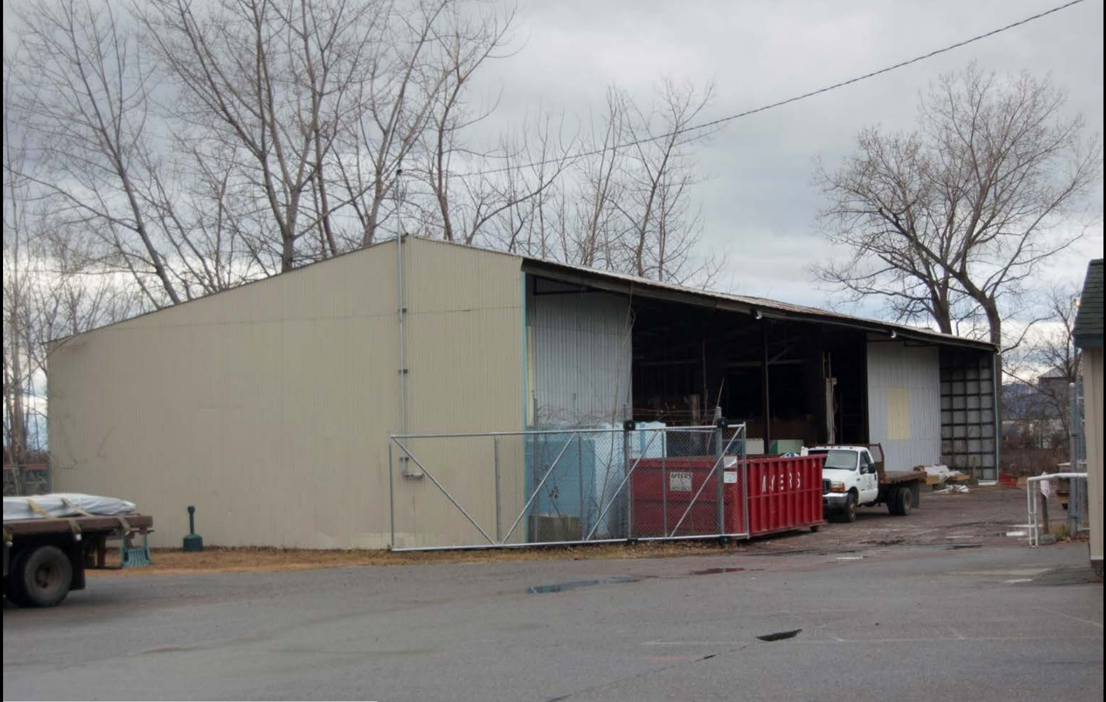
Photo 19. View looking west at HD #9b Lumber Shed.
