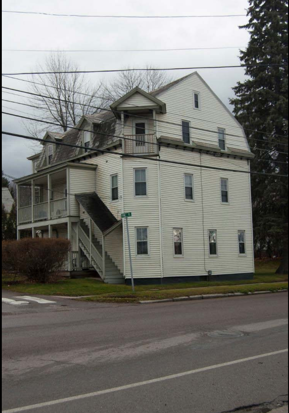
Photo 30. View looking southeast at HD #14 Meunier Store/Glove Factory/Dwelling.
