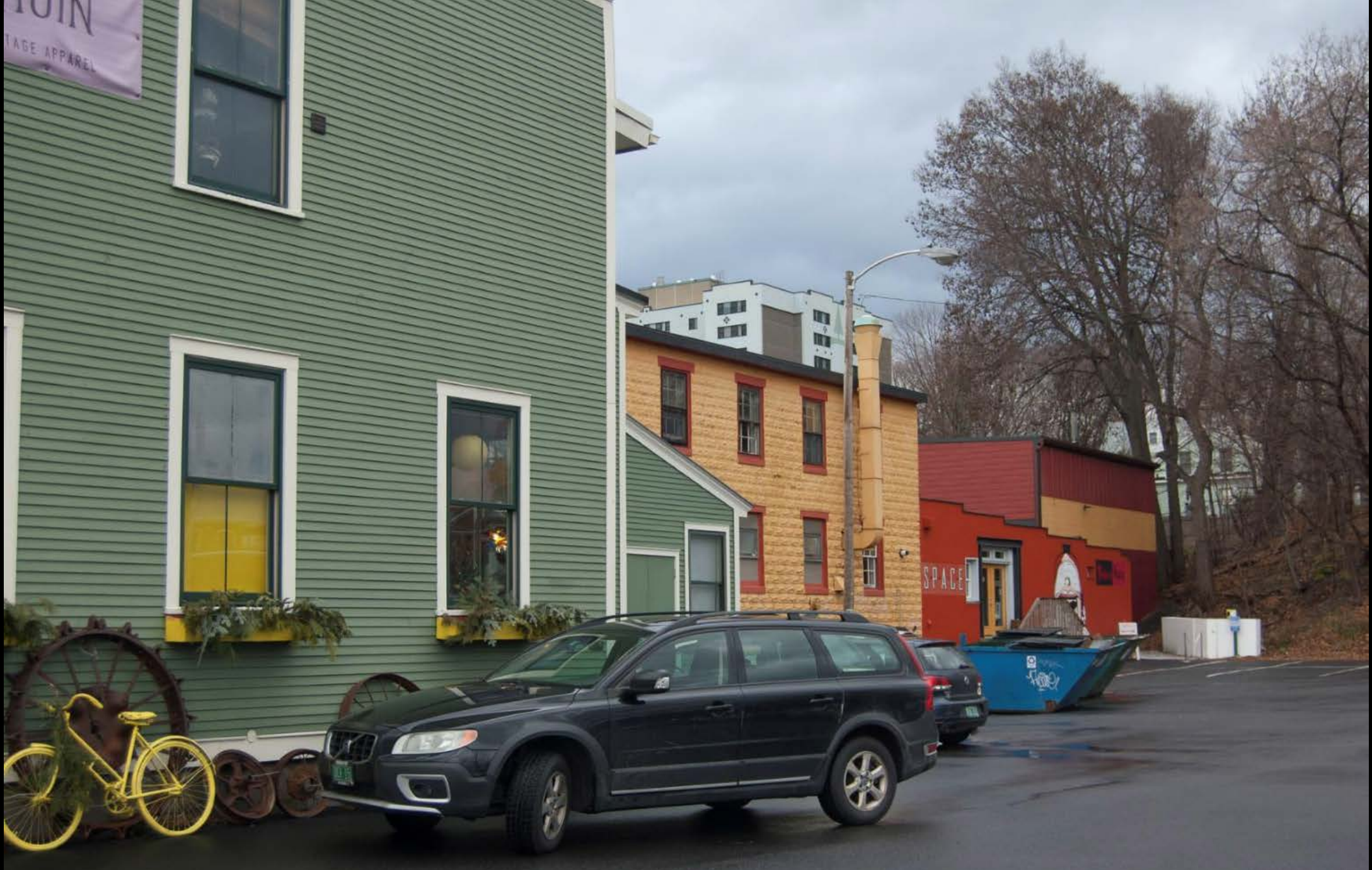
Photo 32. View looking northeast at south wall of HD #8 Burlington Venetian Blind Company Office (left) and rear of HD #7 M. & F.C. Dorn Bottling Works.
