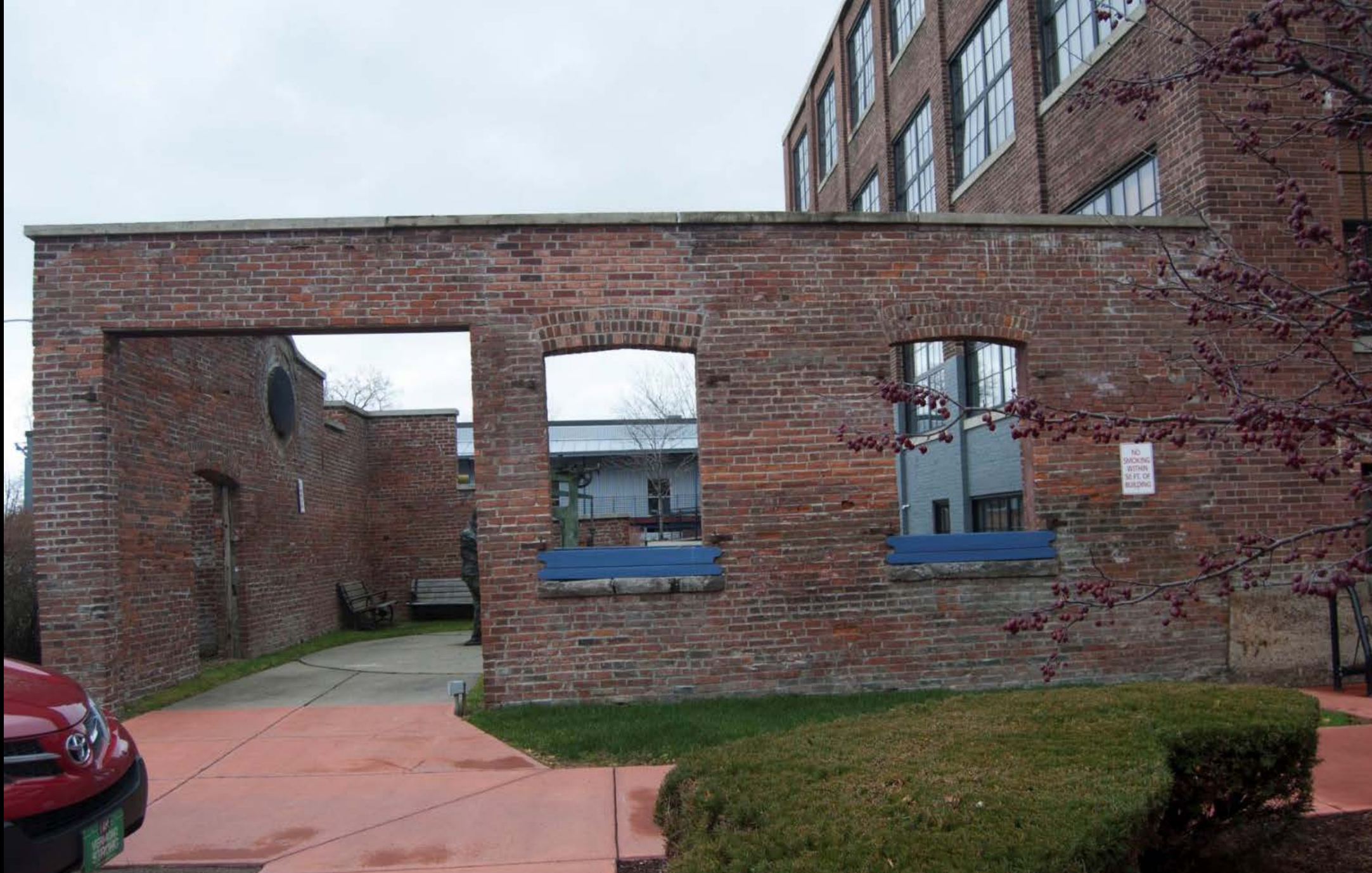
Photo 44. View looking north at HD #19 Malted Cereal Company.
