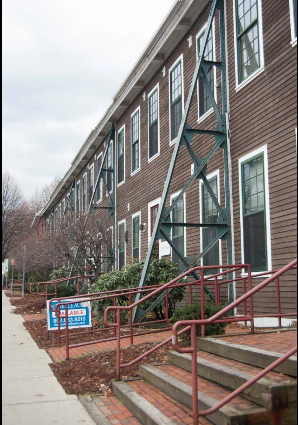
Photo 24. View looking east along north wall of HD #11 Kilburn and Gates.
