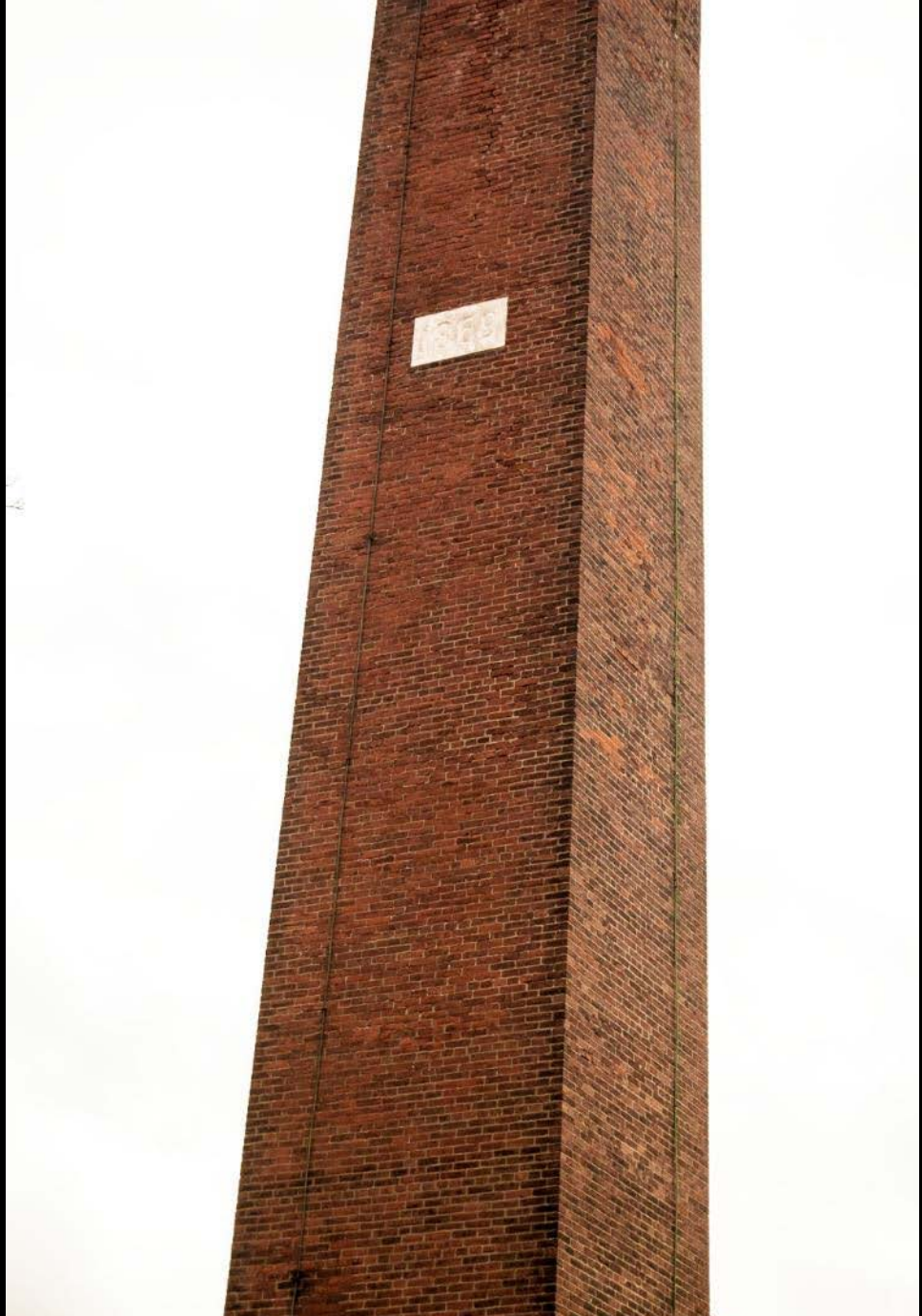
Photo 26. Detail of "1869" date block on chimney at HD #11 Kilburn and Gates.
