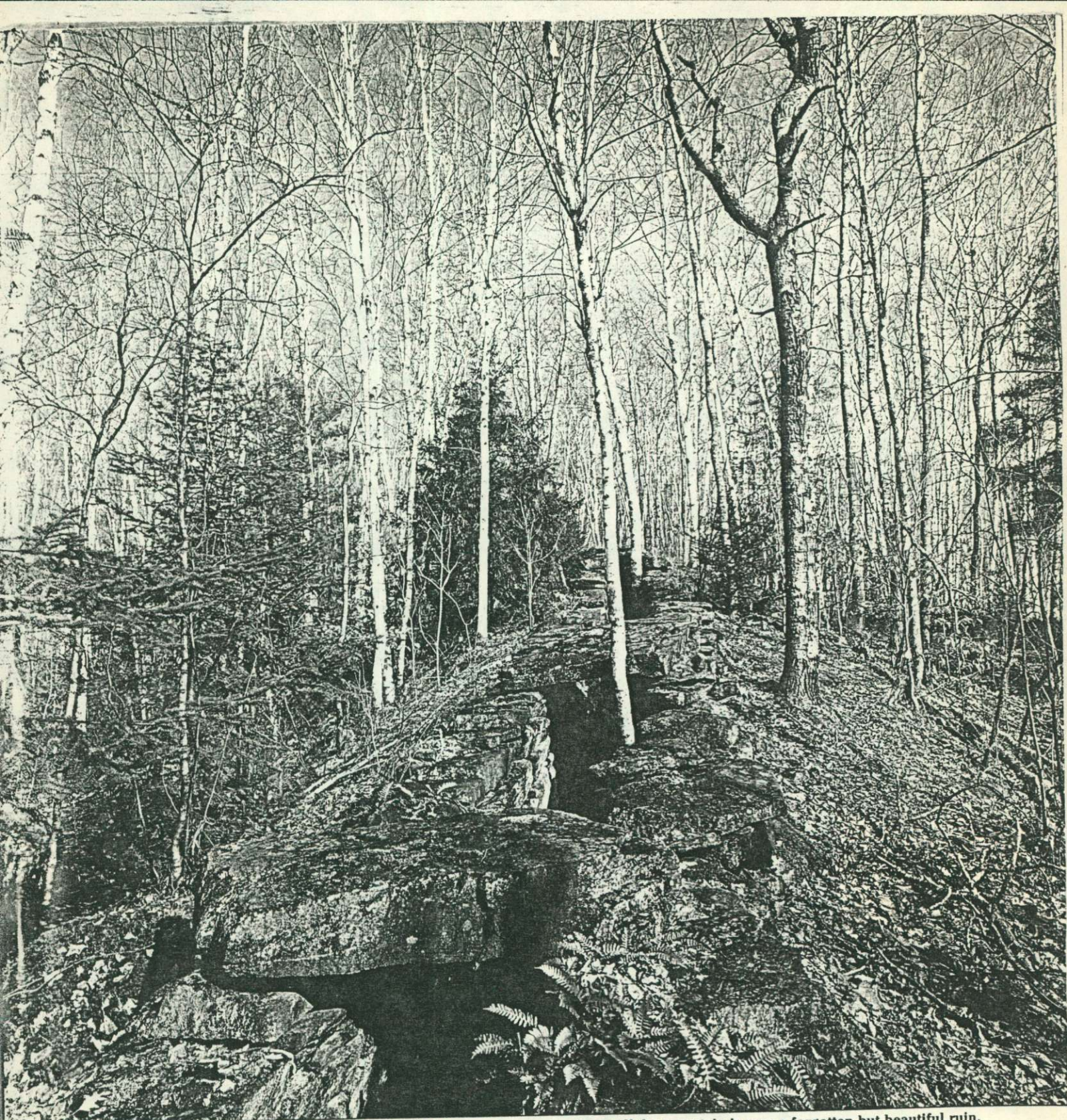
The six-foot-deep stonework trench that carried the copper mine's smoke up off the mountain is now a forgotten but beautiful ruin.
