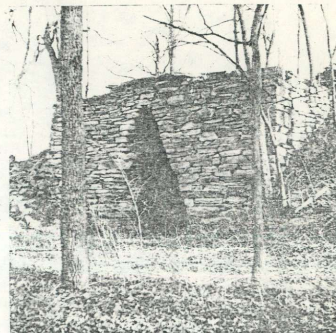
Limekiln with triangular opening. Located on farm near Sheridan, Berks County.
