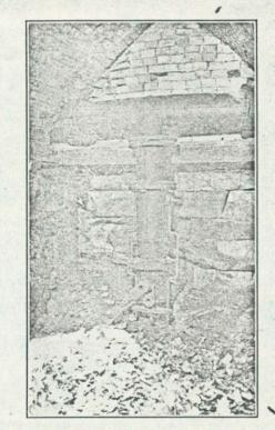
Bustle-pipe, dropper, and tuyere stock for rear tuyere, Sharparoon furnace. Note peep-hole and cover, damper stem where clamping rod is attached, and the sandstone hearth blocks.
