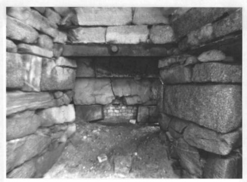
Figure 29. Cross beam inside the south arch.
