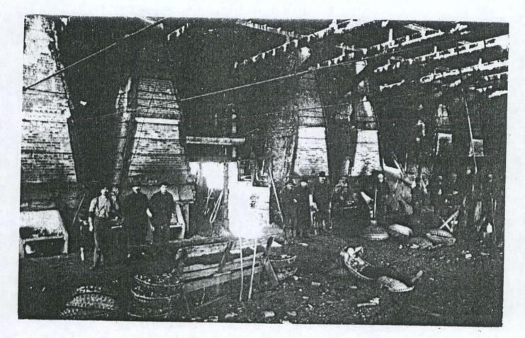
Figure 14. Interior view of the forge at Jay, New York, in 1888, but probably very similar in appearance to that at East Middlebury, Vermont, in the 1880s. Notice that forge hearths were built on the dirt floor. Man at right-foreground is lying in a charcoal basket (courtesy Adirondack Museum).
