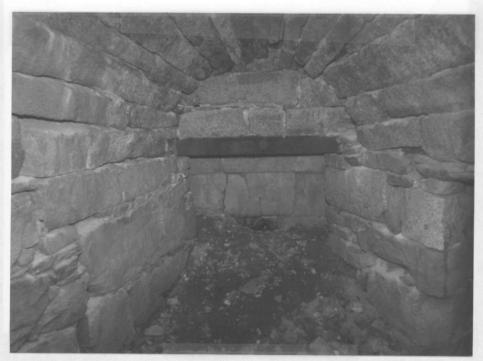
Figure 30. Cross beam inside the west arch.
