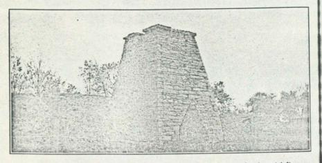
Beekman steam-blown furnace with top of oven on ground just showing at left.
