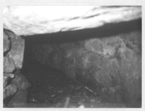
Figure 44. Inside the tunnel, taken by holding a flash camera just inside the small opening. Note the stone wall in good condition.
