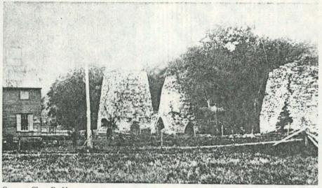
Bennington Iron Works furnaces as they appeared about 1870. The center, smaller stack was called the "Pup." Ironmaster Thomas Trenor burned down a predecessor to one of these furnaces, mistakenly charging it with manganese instead of iron.
