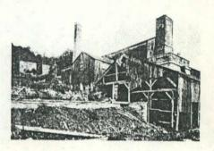
Figure 4. The steel works at Roxbury in the 1890s. The roasting furnaces may be seen in the background. The blast furnace with its brick stack is at the right. Courtesy of Robert Gordon.
