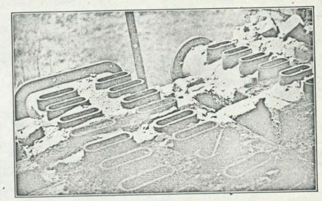
Maltby furnace manifolds in oven floor. Note flue openings between, up which hot gases came.
