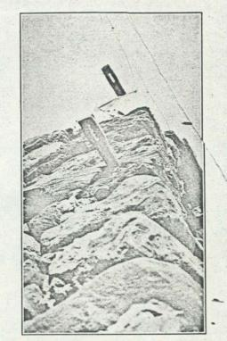
Corner of Mi. Riga furnace. Note timber tie beams, slotted . tie rods, and rough character of masonry.
