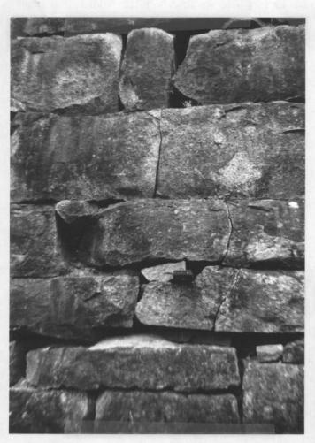
← Figure 11. Hairline cracks in the otherwise solid masonry of the northeast pillar wall,
