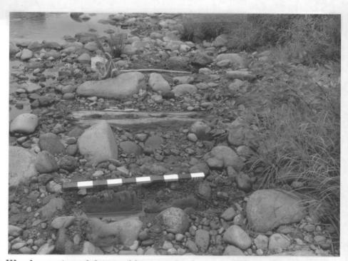
Figure 41. Wood remains of dam cribbing at the dam site (Megan Battey photo).
