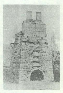
Circa 1900 view of the stack's north wall before it collapsed. Note the blast heating oven at the top.
