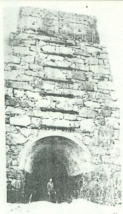
Blast furnace built at Tahawus about same year as Sisco. It was 48 ft. high whereas Sisco stood about 60 ft. The involved a furnace ers. One man, Sr. down his masonry.
