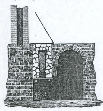
Figure 7. A cast steel air furnace showing the crucible in place in its compartment (left, center) under the door (Overman 1850:476).
