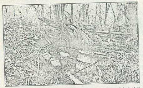
Kent furnace blowing machinery today. Note tail-rod extending from cylinder-head of tub, the relief holes at top of equalizer (in the foreground), and the water-wheel shaft and spiders in background.
