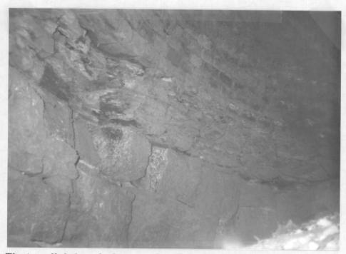
Figure 34. The inwall, below the bottom edge of the furnace lining, just above the north arch. Large inwall stones have fallen from the holes at left, encouraging lining bricks above to drop down.
