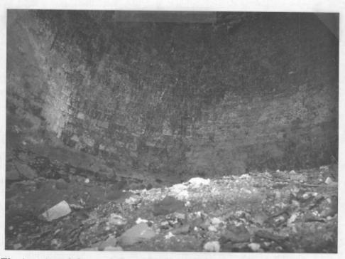
Figure 33. The interior of the stack from the access hole inside the west arch, looking eastward across the top of the mass of breakdown atop the hearth.
