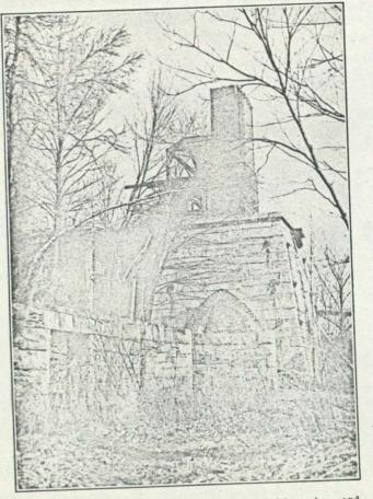
Roxbury furnace. Note fine ashlar masonry, brick arches, and heavy wall plates at ends of tie rods.
