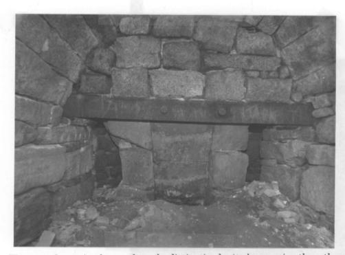
Figure 25. The cross beam in the north arch, distinctive by its larger size than those in the other three arches.
