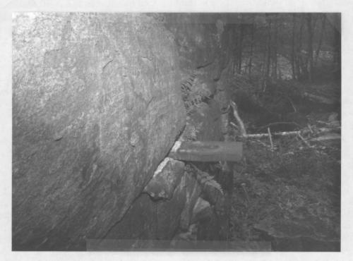
Figure 22. The end of a binder rod sticking out through the southwest pillar wall.
