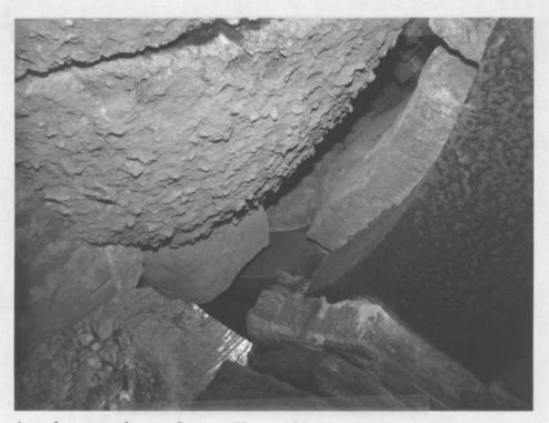
Figure 32. Area between the northeast pillar and bosh, showing how the east arch cross beam ring (right) misaligns with its counterpart in the north arch.
