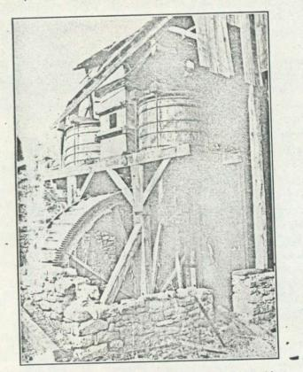
Hopewell furnace (Pennsylvania) blowing machine, with square wind-box or equalizer between tubs. Courtesy Mr. Lewis Dalrymple Bradbury
