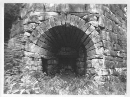
Figure 18. The east arch, showing the downer pipe (right), the cross beam with one knob (center), and the passageway to the south arch (left).
