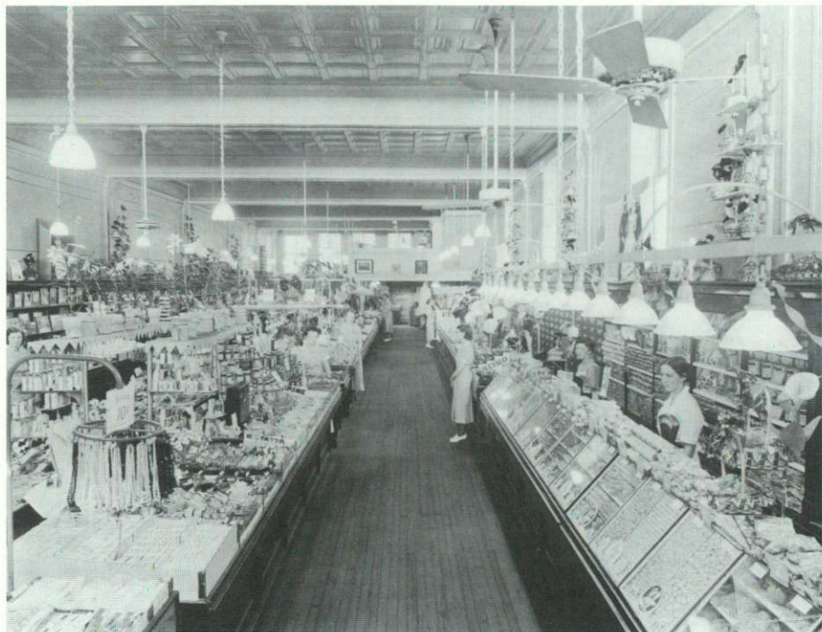
Anderson, South Carolina
