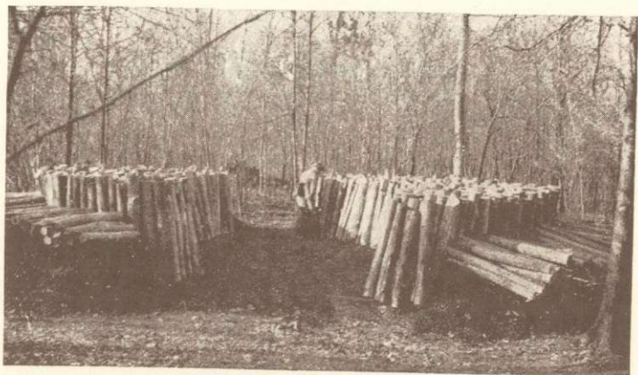
Filling a hearth with lap-wood and billets
