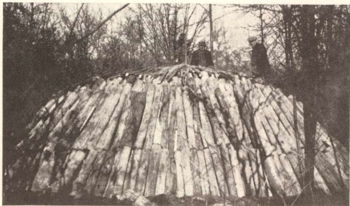
Pit ready for covering
