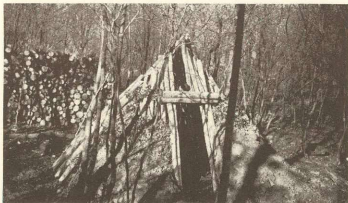
Collier's hut under construction
