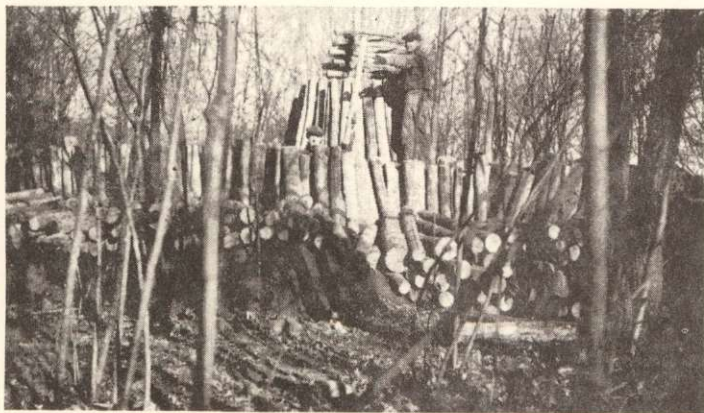
Constructing the chimney
