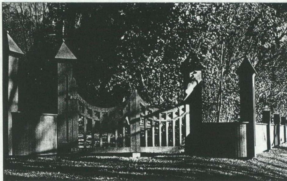
Builder Blake Spencer used historical photos to work out the details of the historic fence restoration at the Morrill Homestead in Strafford, Vt. The main gate is the kind you would imagine passing through on the way to meet St. Peter. Or Walt Disney.
