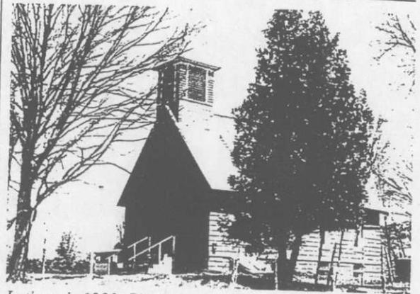
*In the early 1900s Pittsford marble workers constructed this chapel (11), convenient to their homes around the Florence area quarries. This building is rather unusual because, although the roof is covered with local slate, the walls are built of man-made pressed stone blocks instead of marble.*
