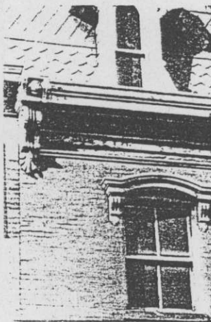
Illus. 5. The four historic examples of various window hoods shown are: (a) stone; (b) cast stone; (c) cast-iron; and (d) sheet metal. The criteria for selecting substitute materials today (availability, quality, delivery dates, cost) are not much different from the past. Photo: Sharon C. Park, AIA.
