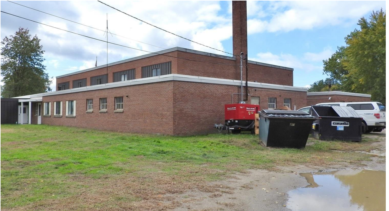
12. Facing southwest toward east and rear/north elevations
