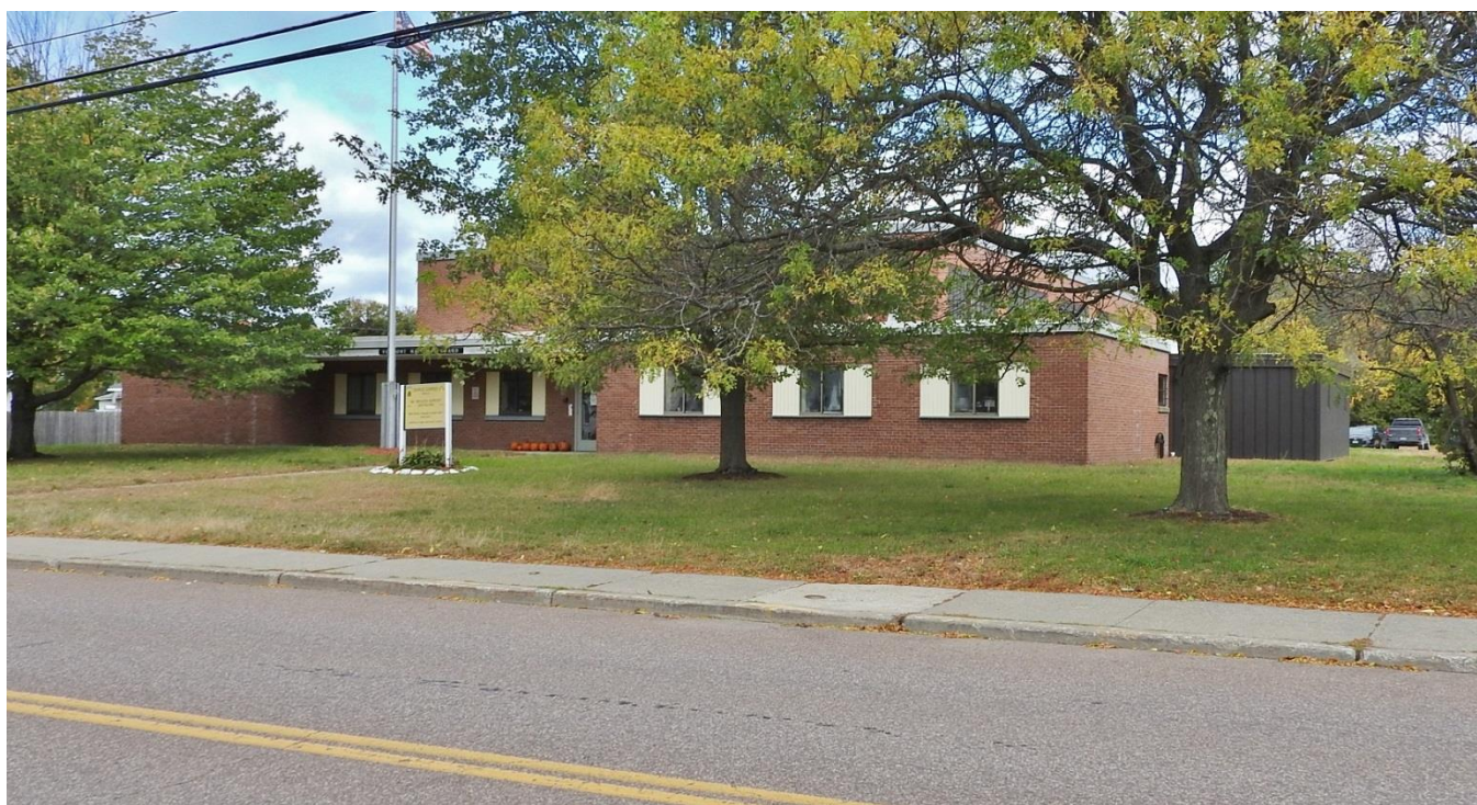
2. Facing northwest toward front/south elevation
