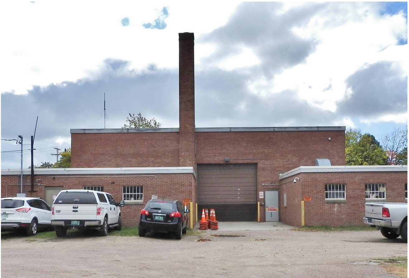
15. Facing south toward rear/north elevation
