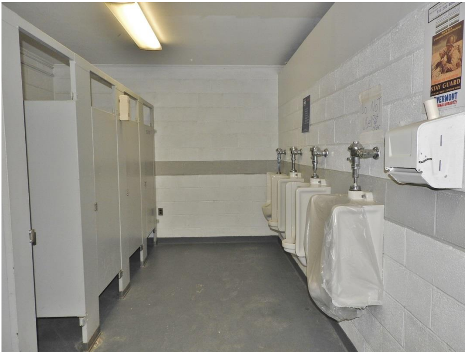
29. Facing north in men's latrine
