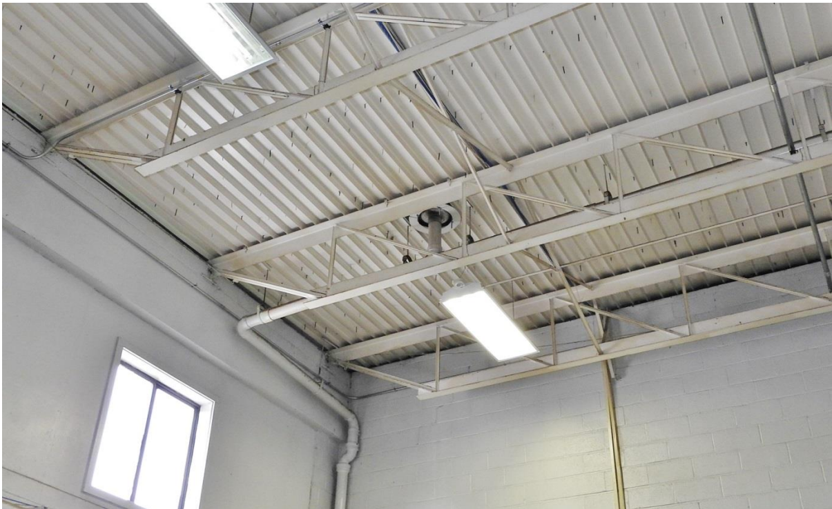
26. Detail of drill hall roof structure
