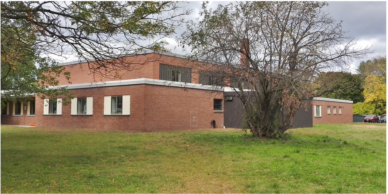
5. Facing northwest toward south and east elevations
