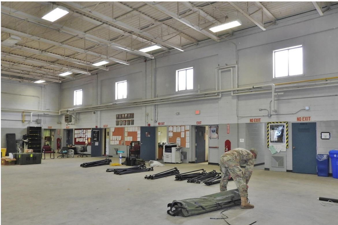
24. Facing northeast in drill hall
