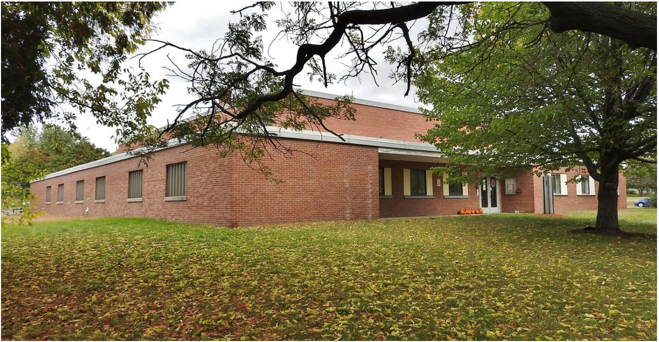
7. Facing northeast toward west and front/south elevations
