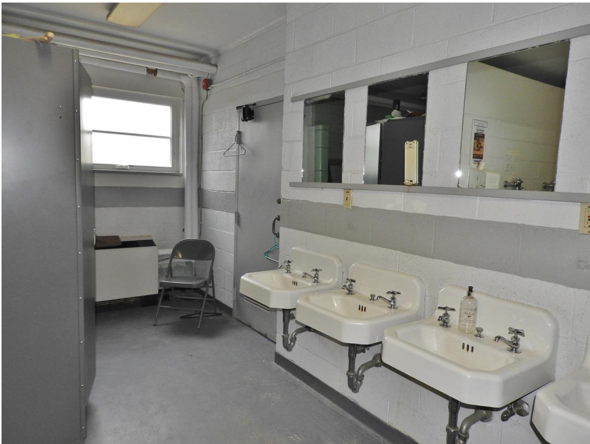
28. Facing east in men's latrine
