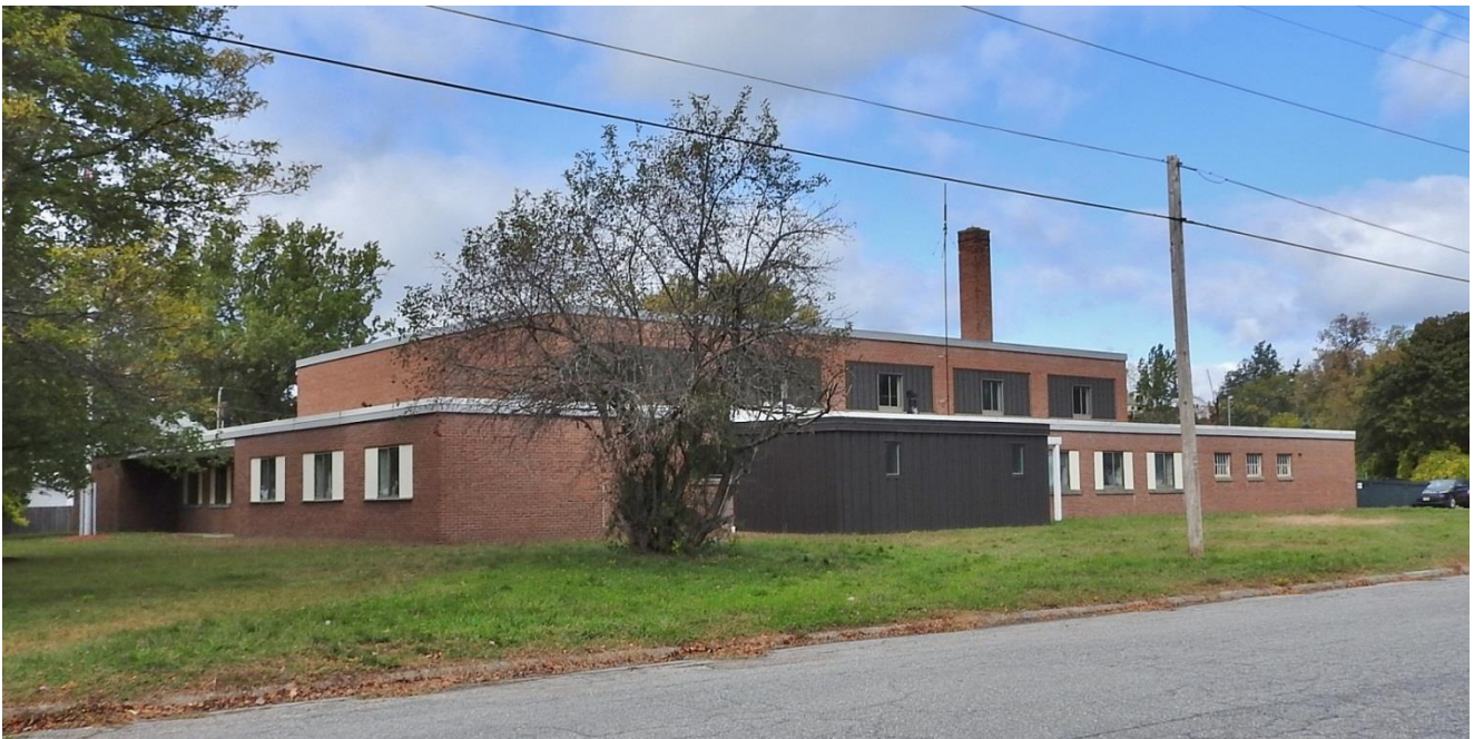
4. Facing northwest toward south and east elevations
