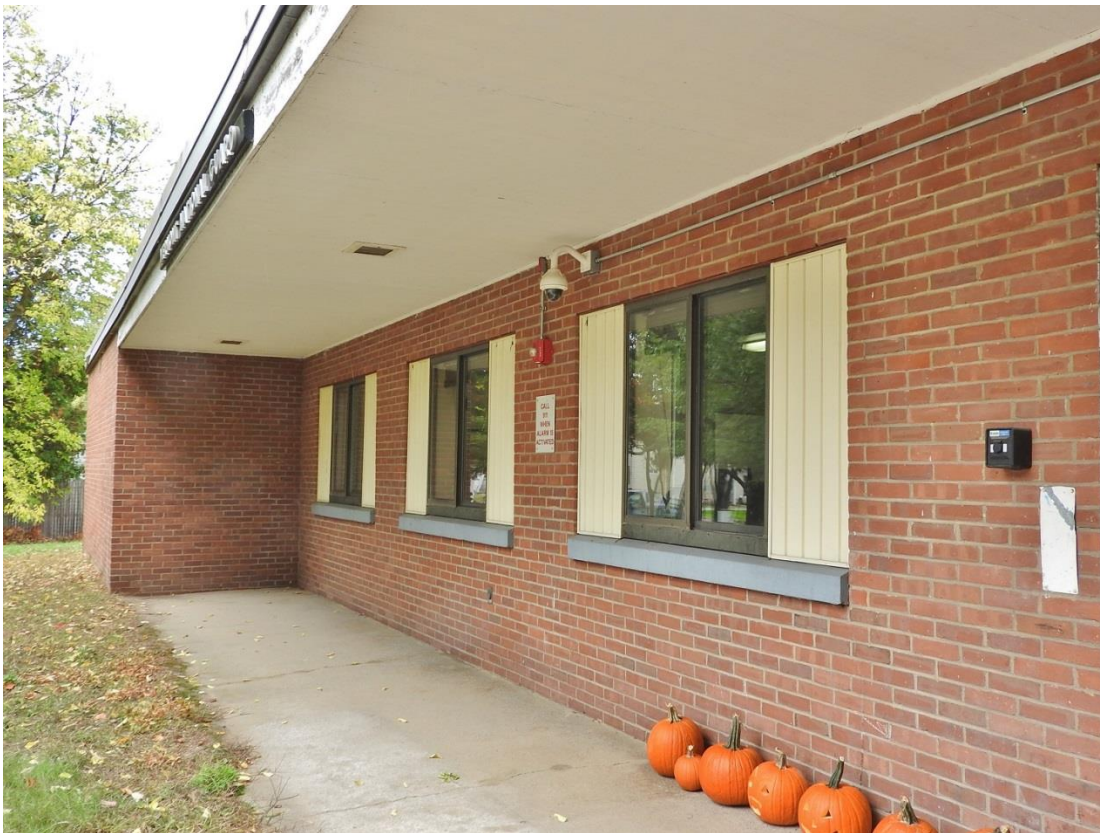
10. Facing west toward front porch
