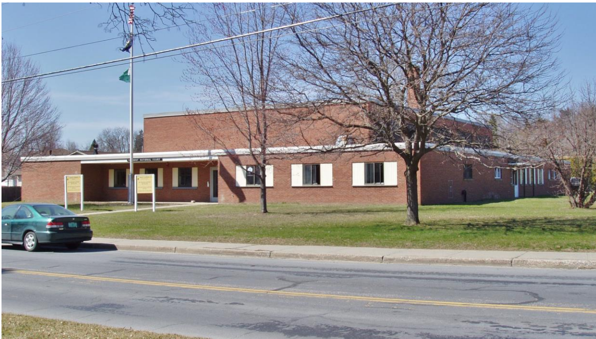
40. Facing northwest toward front/south and east elevations, 2009.
