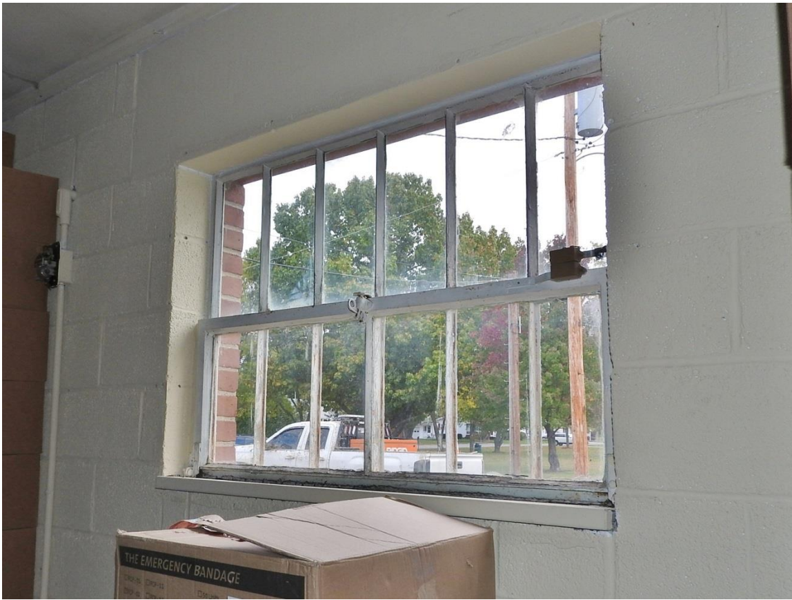
35. Original window at east elevation
