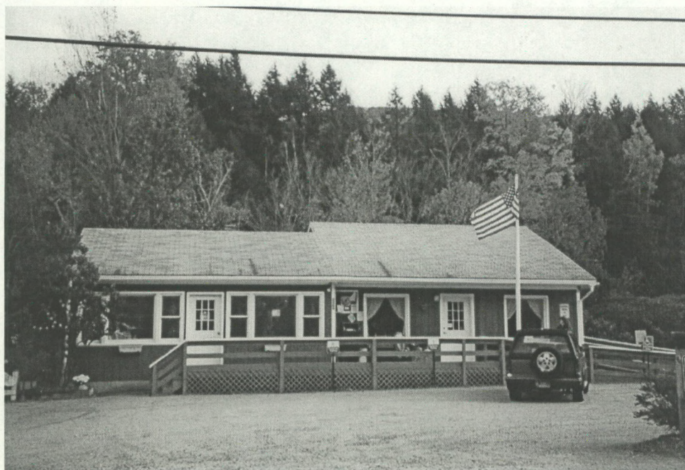
Brownsville Post Office façade Photographer facing: S
