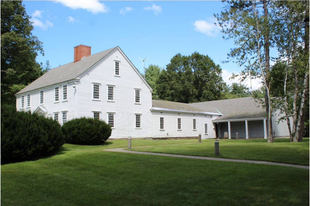
Photo 2: Vermont_Windham_GovernorHuntHouse_0002: ¾ shot of the façade and southern elevation of the 1779 portion of the house as well as the rear additions built by Vermont Yankee. Camera facing north.
