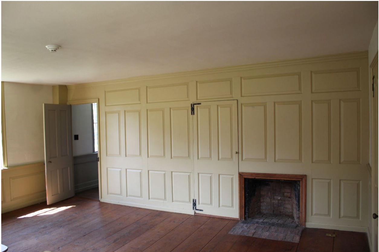
Photo 13: Vermont_Windham_GovernorHuntHouse_0013: Second story children's bedroom showing fireplace and paneling. Camera facing north.
