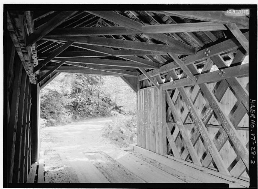
BROWN BRIDGE. Interior, northeast portal. Photograph by Jet Lowe, 2004 [HAER VT-28-2]
