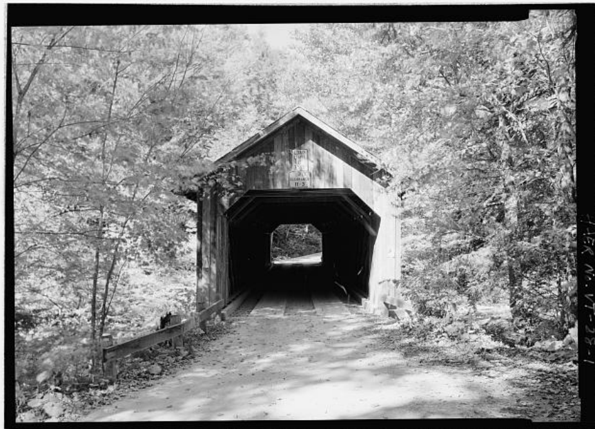
BROWN BRIDGE. Northeast portal. Photograph by Jet Lowe, 2004[HAER VT-28-1]
