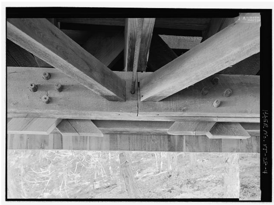
BROWN BRIDGE. Lower chord details. Photograph by Jet Lowe, 2004 [HAER VT-28-4]
