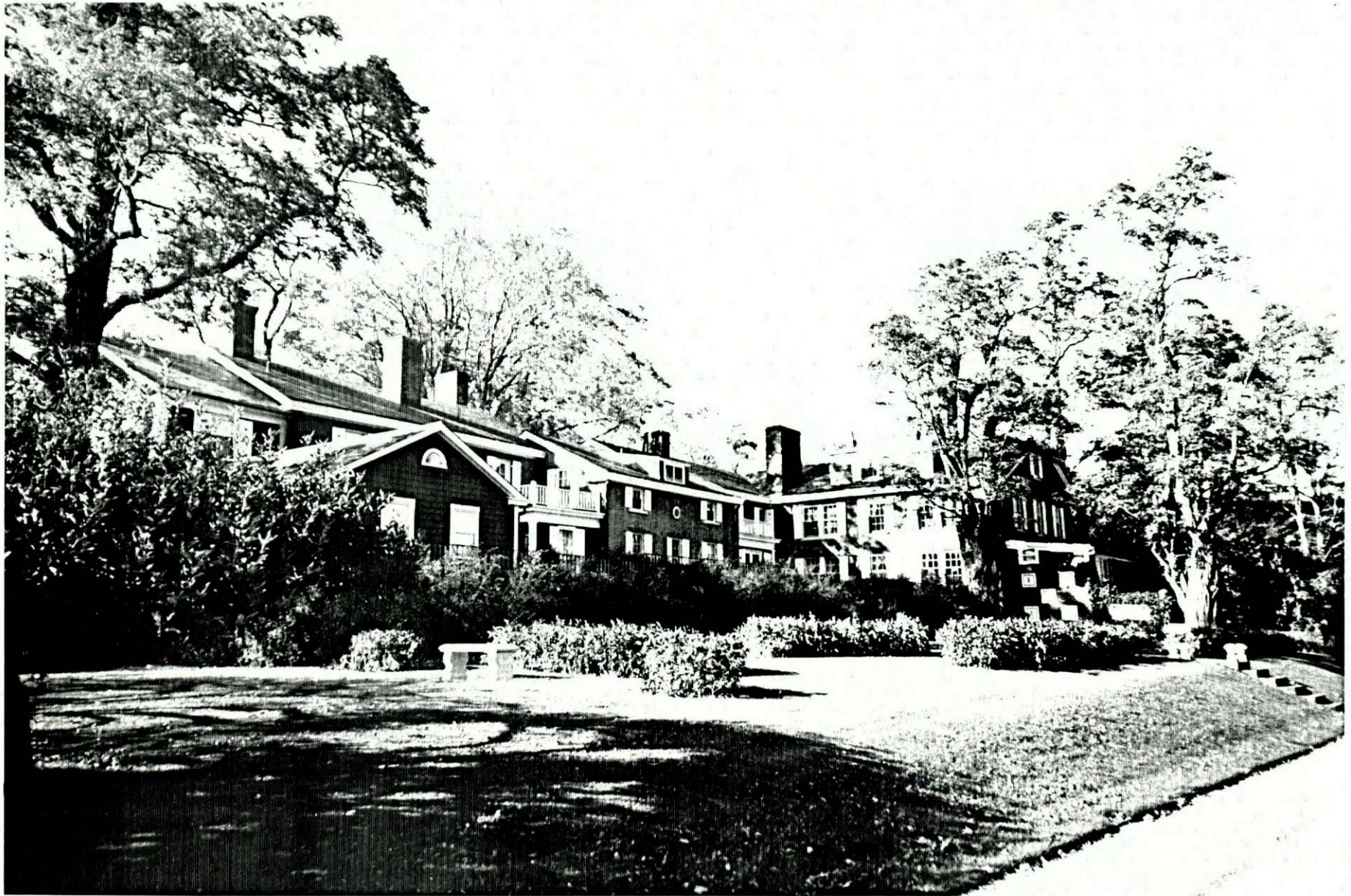
Brick House, Shelburne, Vermont East facade - view looking northwest Credit: E. Wadhams 10/97
