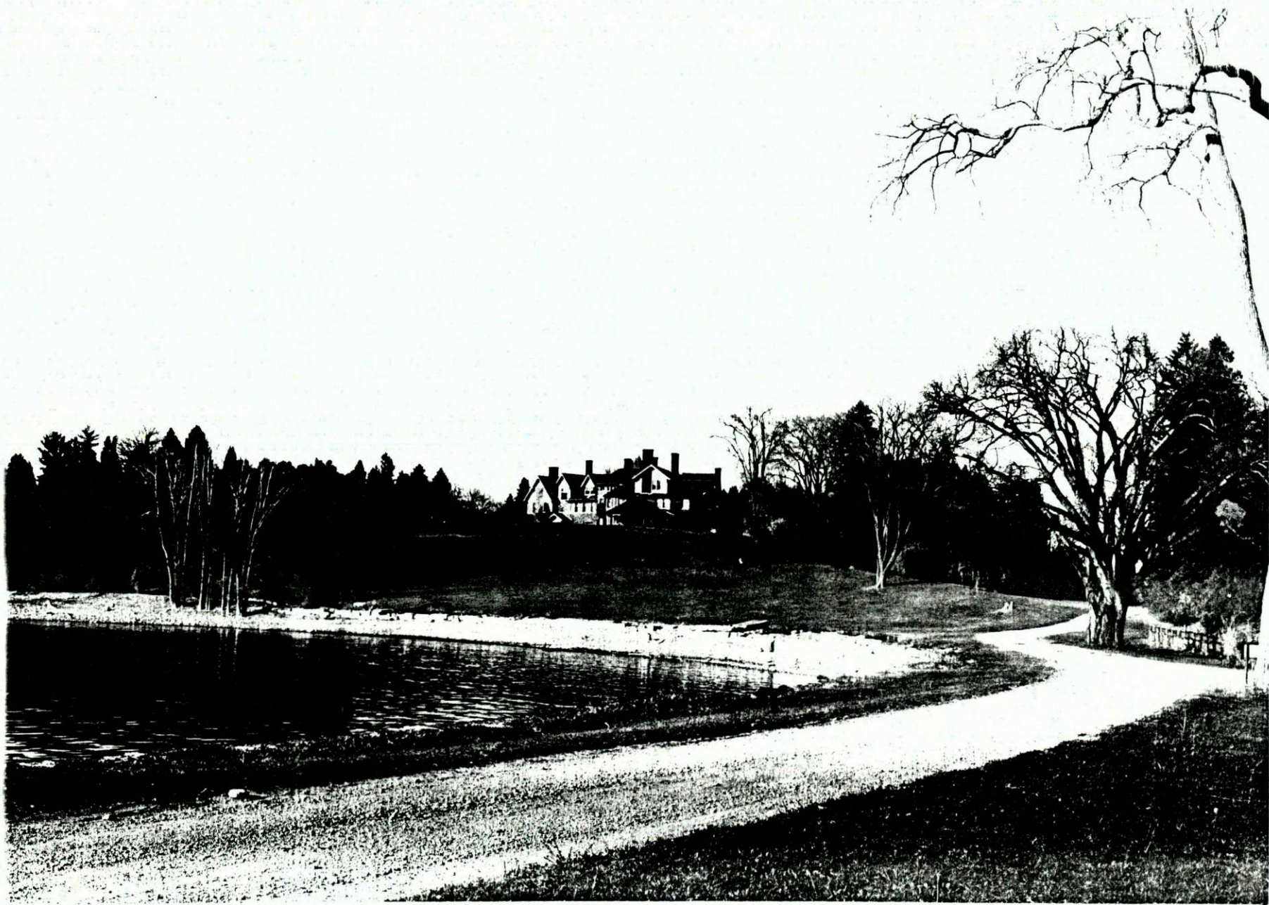
Shelburne Farms Shelburne, Vermont Shelburne House from road Photo: John Dumville, 1978
