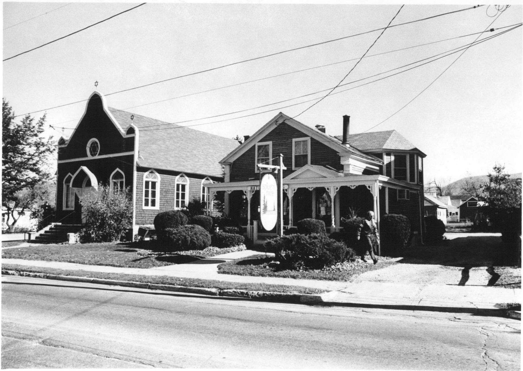
223, 225 North Street NE 88-A-264 Tracy Cuning VT Division for Hist. Preservation Bennington Co. Bennington 10/88
