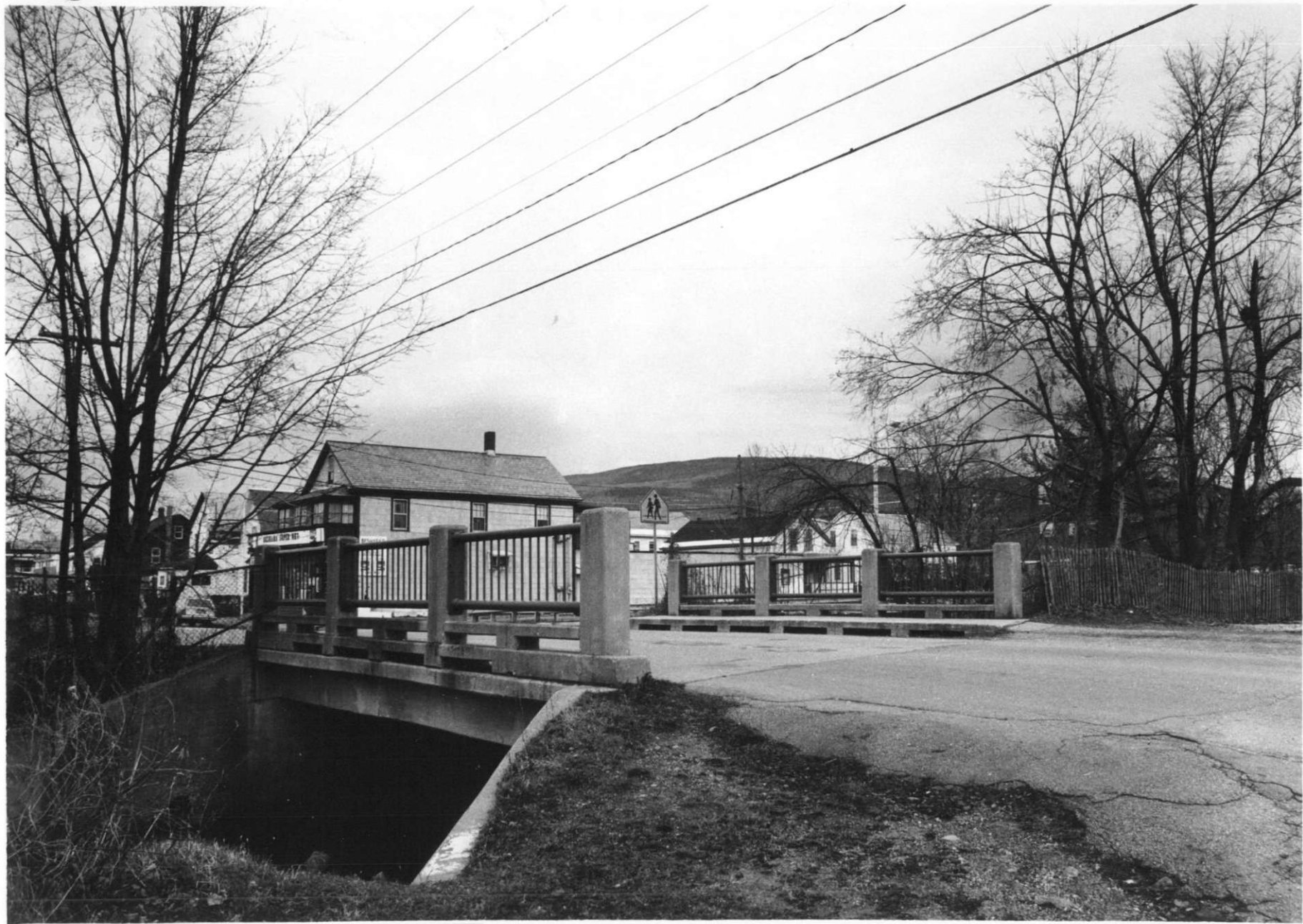
Park Street Bridge NE 88-A-280 Tracy Cuning VT Division for Hist. Preservation Bennington Co. Bennington 10/88
