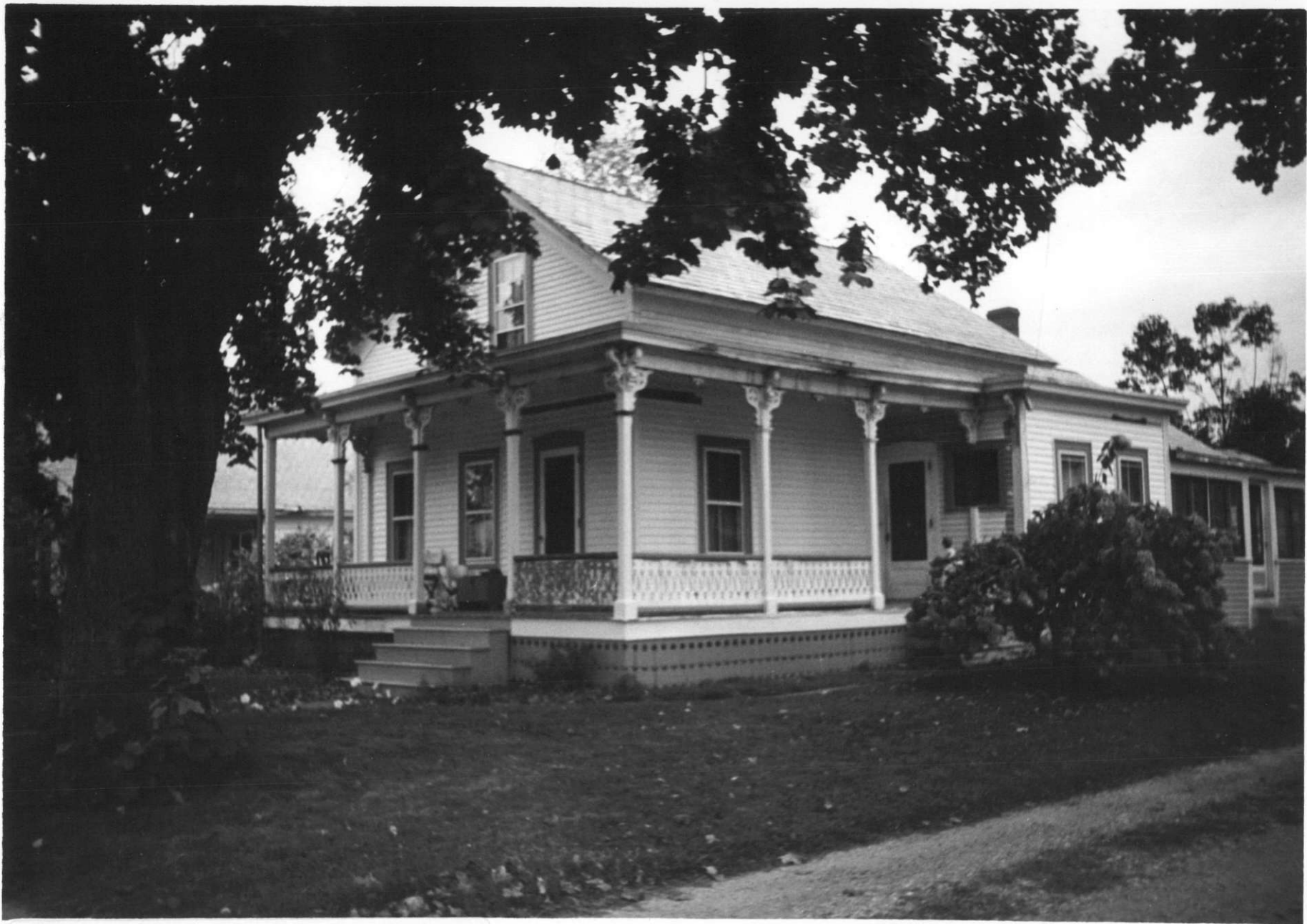
225 Maple Street NE 88-A-246 Daniel Williamson VT Division for Hist. Preservation Bennington Co. Bennington 10/88
