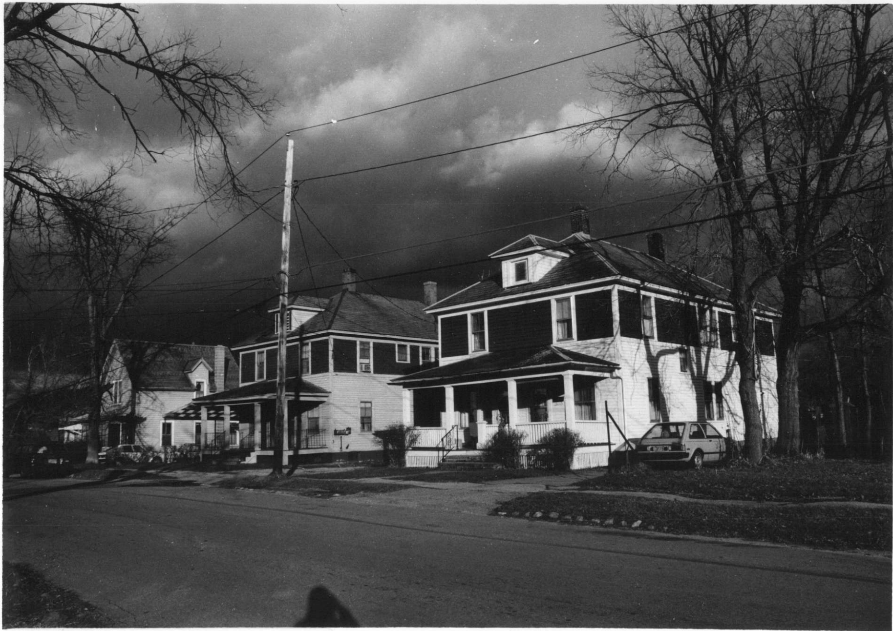
McKinley Street Streetscape NE 88-A-281 Tracy Cuning VT Division for Hist. Preservation Bennington Co. Bennington 10/88
