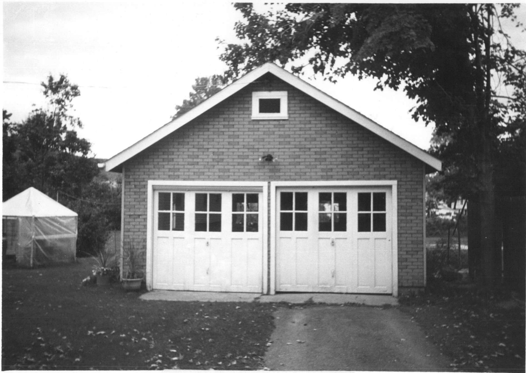
226 Maple Street (garage) W 88-A-246 Daniel Williamson VT Division for Hist. Preservation Bennington Co. Bennington 10/88
