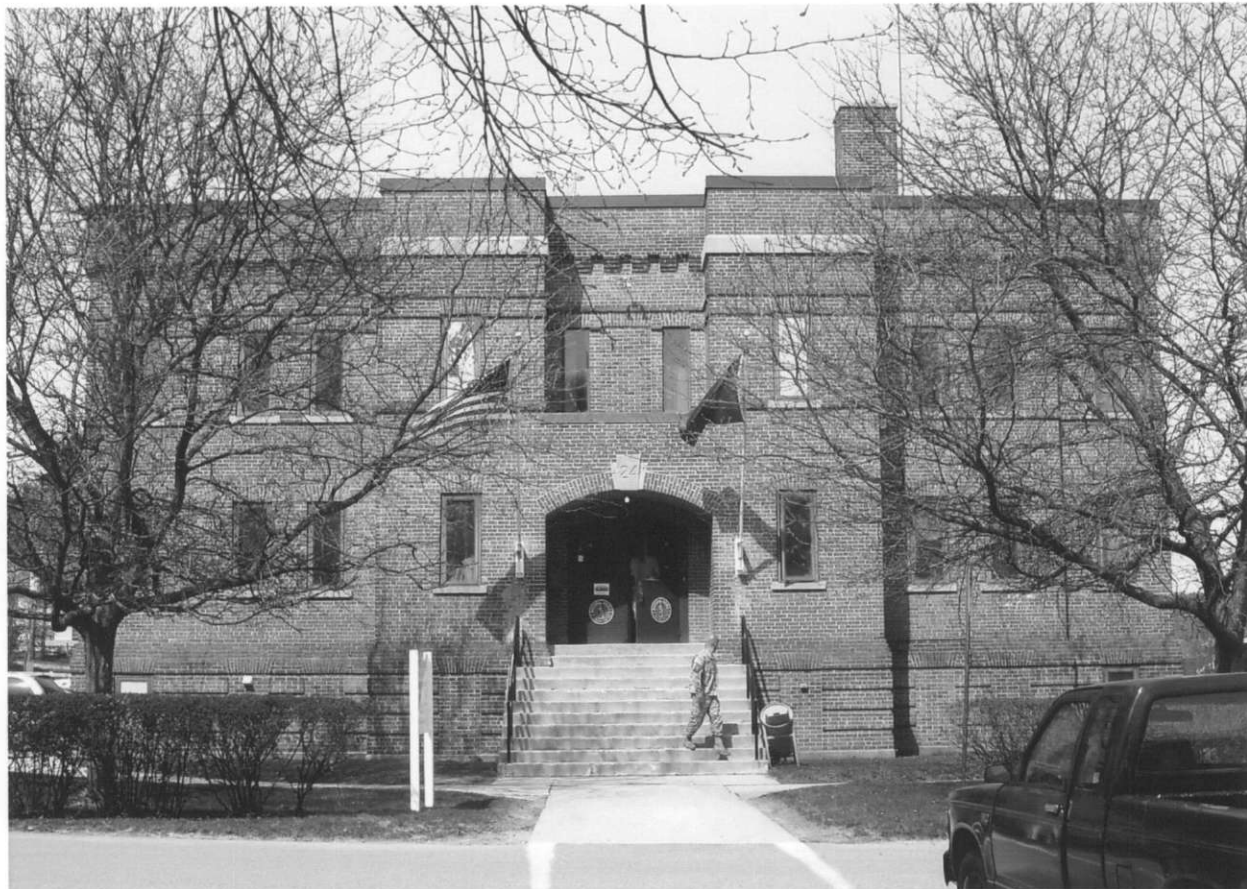
Facing west toward east elevation, July 2009
