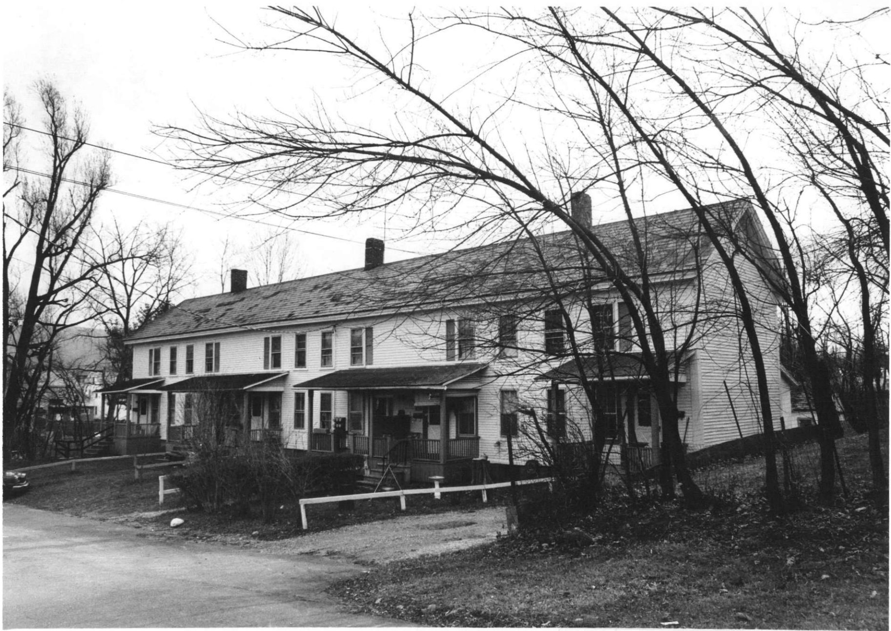
105-115 Holden Street SE 88-A-280 Tracy Cuning VT Division for Hist. Preservation Bennington Co. Bennington 10/88
