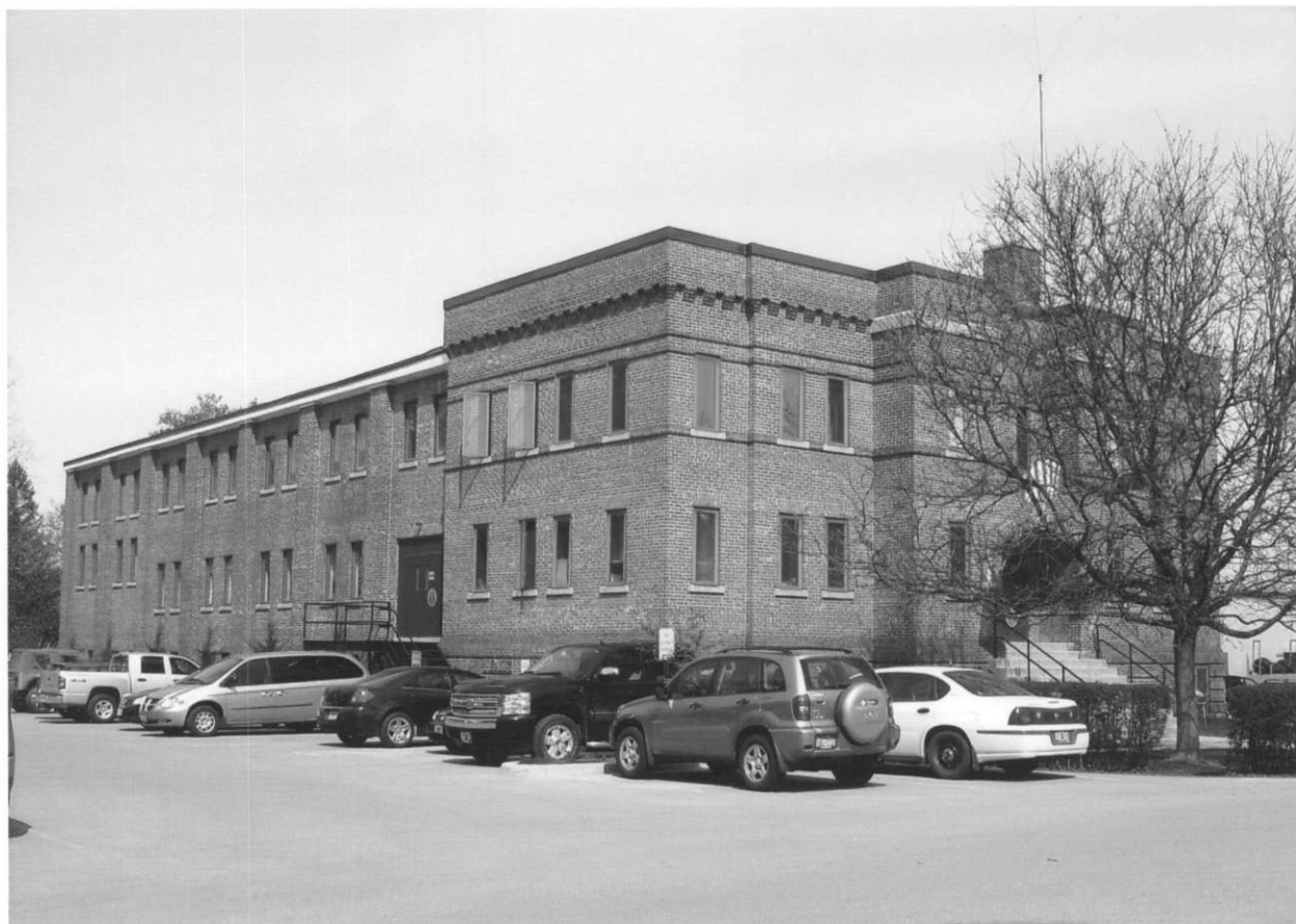
Facing northwest toward south and east elevations, July 2009
